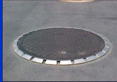
Improve manway lids
