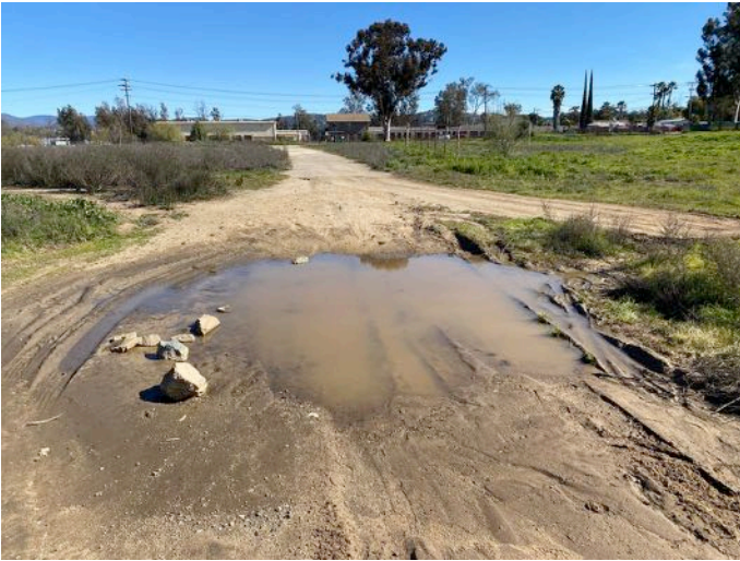
Pool 2 looking northeast.
