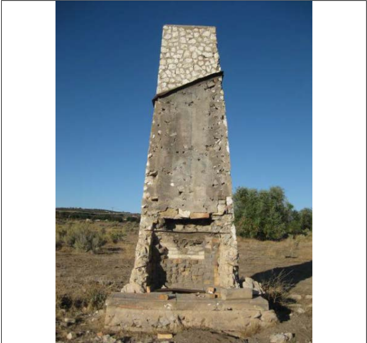
Figure 15 Close-Up of Chimney and Hearth within Site CA-SDI-16824H Feature 1
