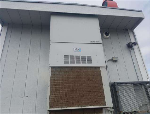
3-Ton Wall Pack AC Unit
