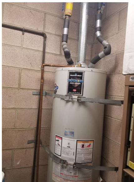
40 Gallon Gas-Fired Water Heater
