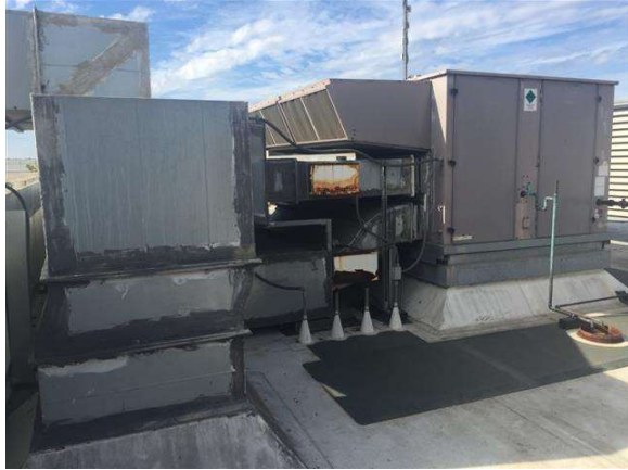
40 Ton VAV Packaged Unit
