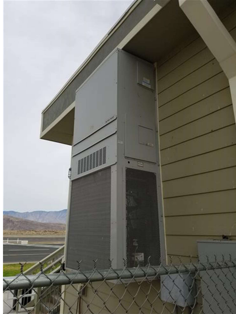
5-Ton Wall Pack Heat Pump
