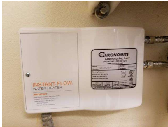
Tankless Electric DWH Heater
