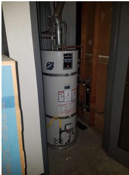
50 Gal Tank-Style Water Heater
