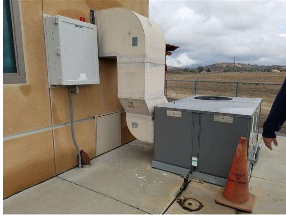
5-Ton Packaged Heat Pump
