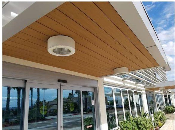
26W CFL in Ceiling-mount Fixture
