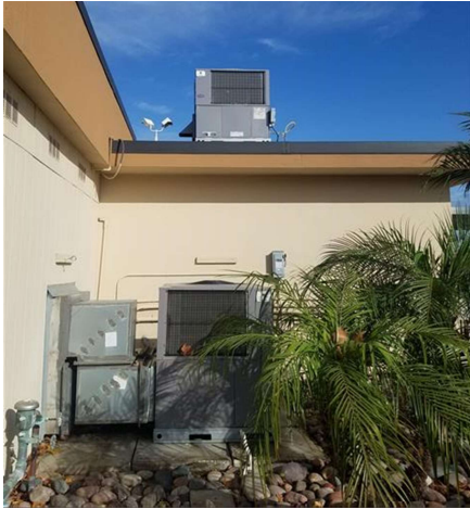
4-Ton Packaged Heat Pump
