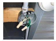
Inspector note: Provide a safety plate for circular junction box located in the mezzanine. Violation is due to be rechecked on 06/01/2021
