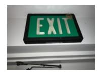
Inspector note: Replace (x2) exit signs due to age. Violation is due to be rechecked on 06/01/2021
