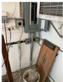
Inspector note: Maintain clearance around the electrical panel. Corrected during inspection.
