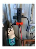
Inspector note: Linking (aka "daisy-chaining") of extension cords, adapters, and power strips is prohibited. Violation is due to be rechecked on 06/01/2021
