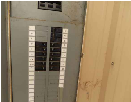
Main Service Hangars "D": Panel Capacity 200 AMP
