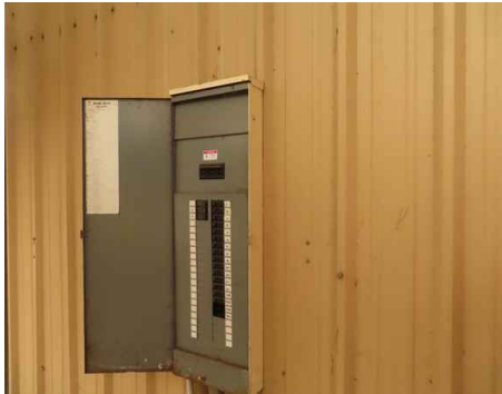
Main Service Hangars "E": Panel Capacity 200 AMP
