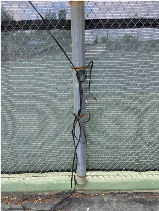
Figure 22 Wiring Concerns
