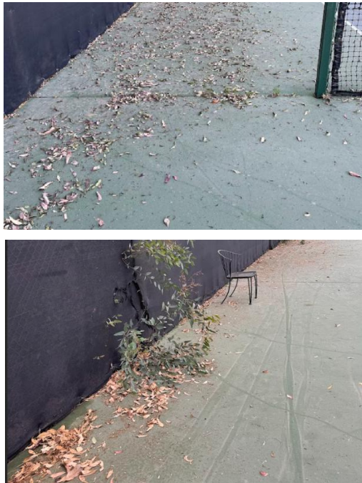
Figure 21 Debris and Leaves Unremoved on Courts
