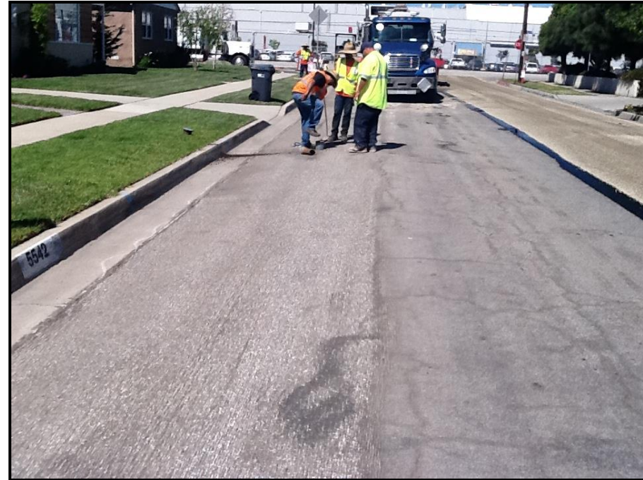
Micro Milled edge flush to gutter face
