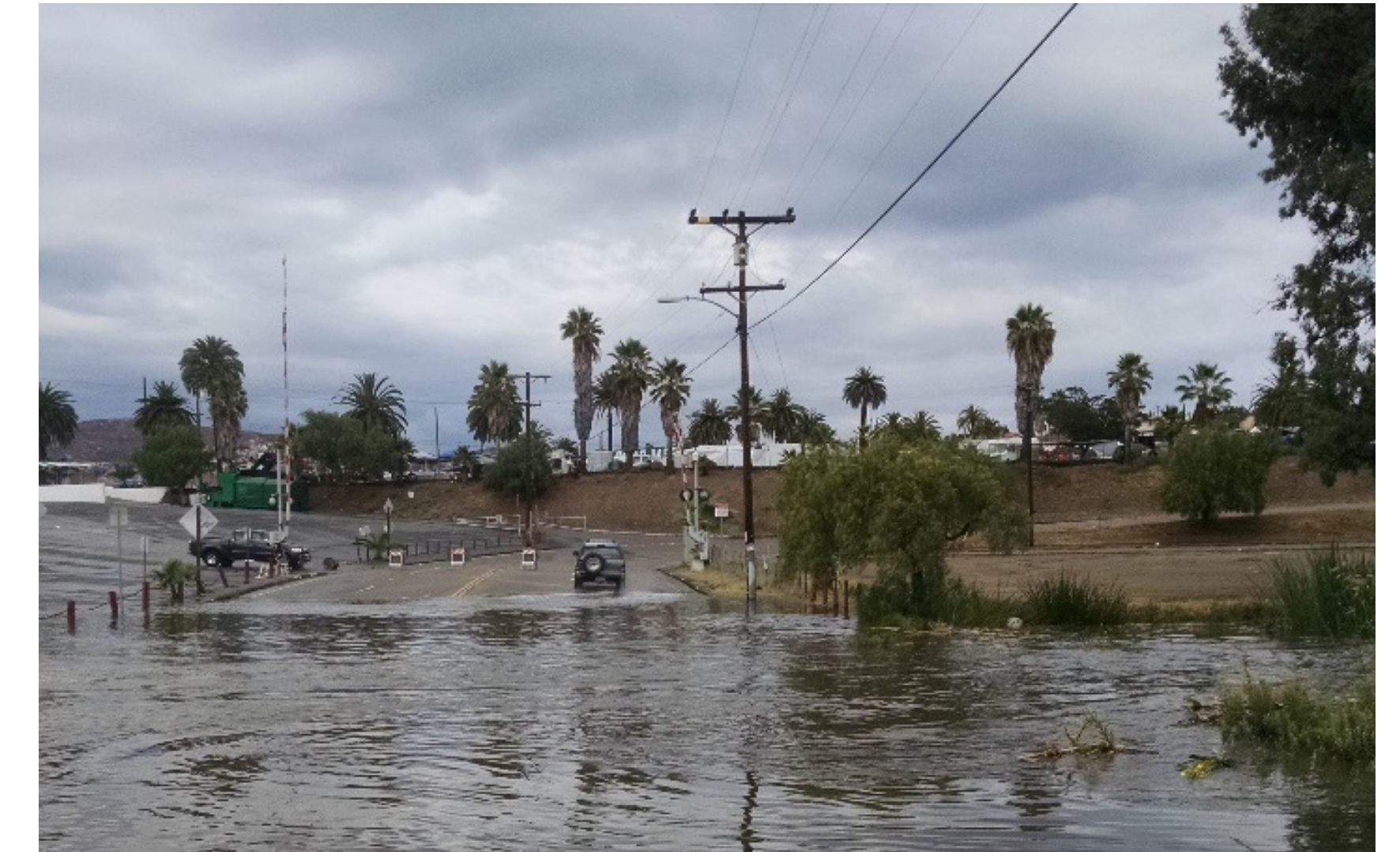
During Flooding Event at Quarry Road
