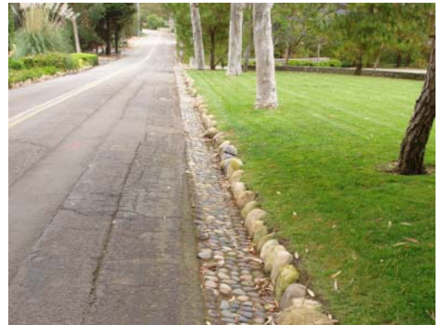
Cobble curb and gutter, 2004
