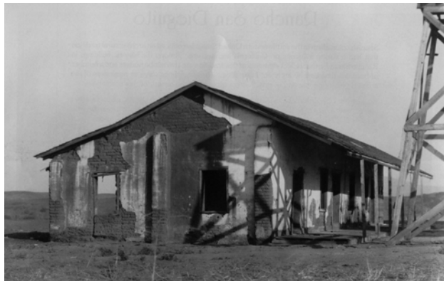
Osuna #1 before restoration
