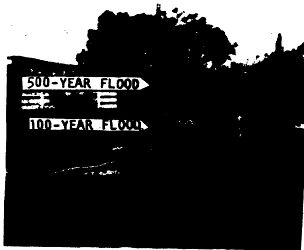
Figure 4. 100- and 500-Year Flood Elevations for Las Puleta Creek at the Delta Street Crossing
