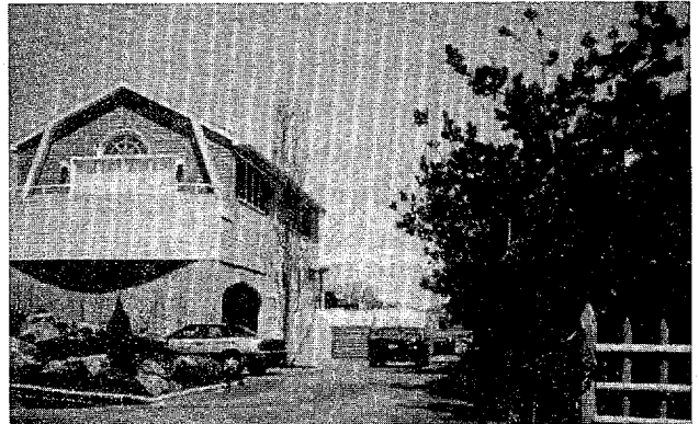
The elevation of this home resulted in the elimination of $25,000 annually in repetitive flood insurance claims. Plantings and berms disguise the retrofit and enhance the landscape.
