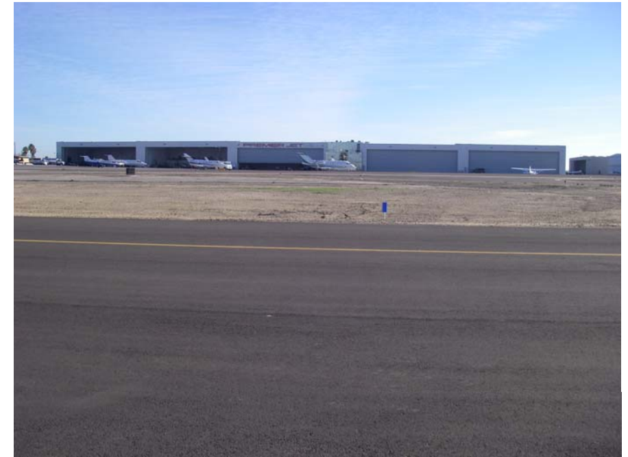
Station 1, January 3, 2007. Looking South
