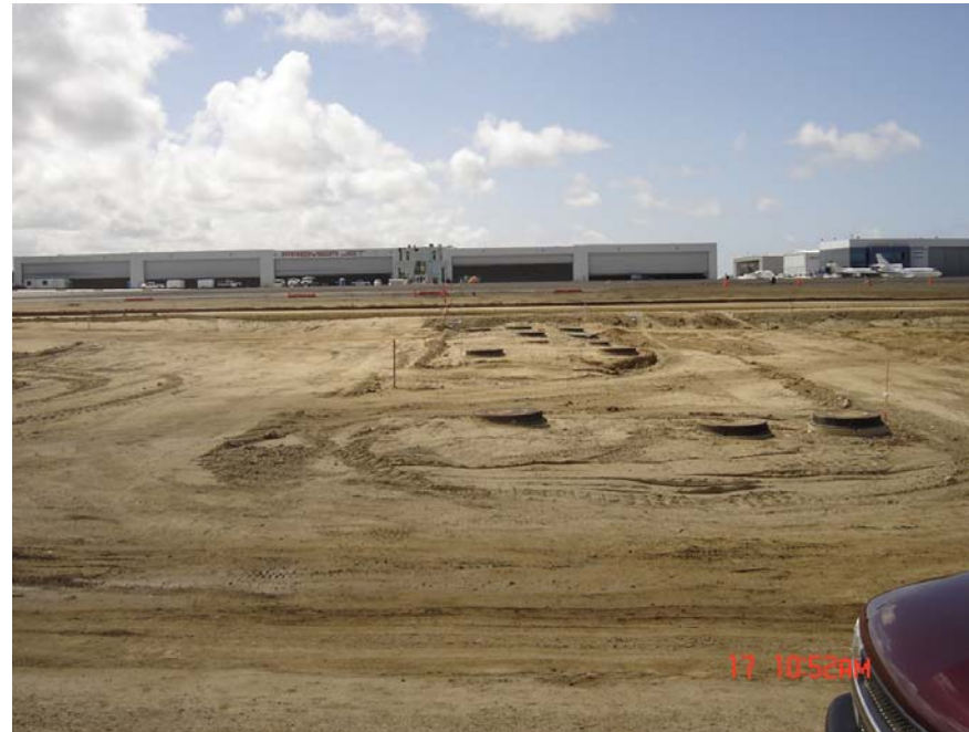
Station 4, April 17, 2006. Looking South.
