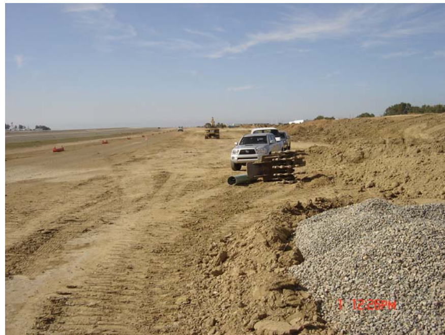
Station 3, February 1, 2006. Looking West.
