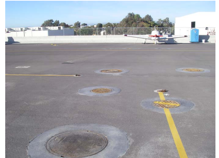
Station 1, January 3, 2007. Looking North
