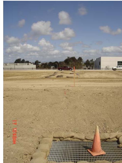
Station 3, April 17, 2006. Looking North.
