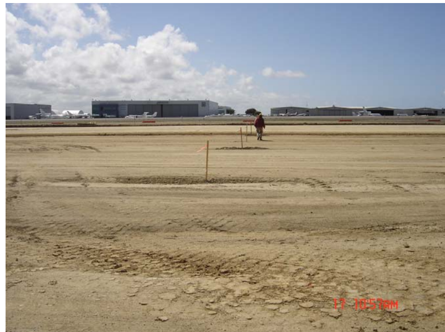
Station 5, April 17, 2006. Looking South.
