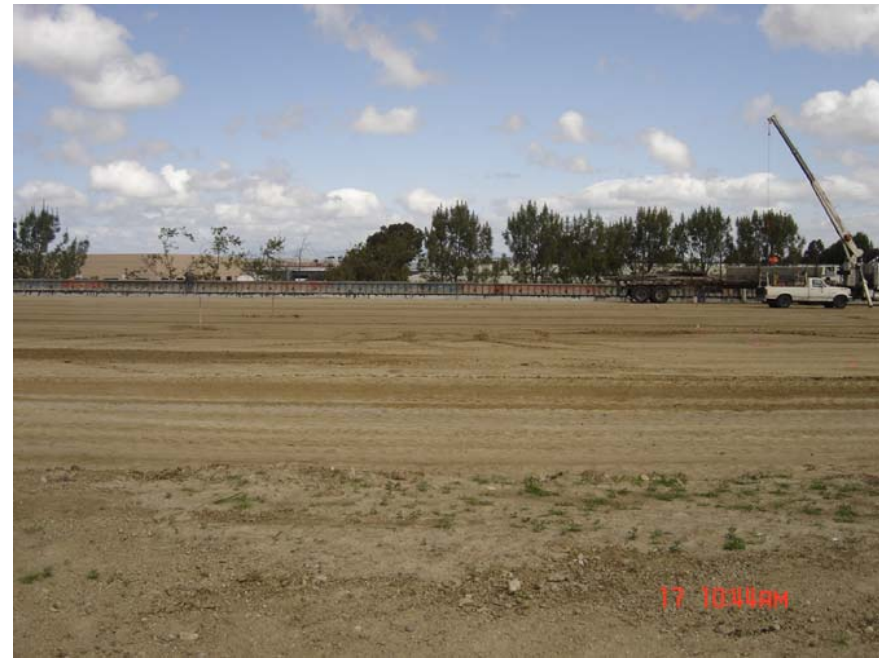
Station 6, April 17, 2006. Looking North.
