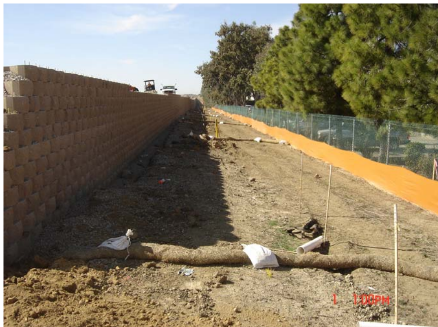
Station 8, February 1, 2006. Looking West.
