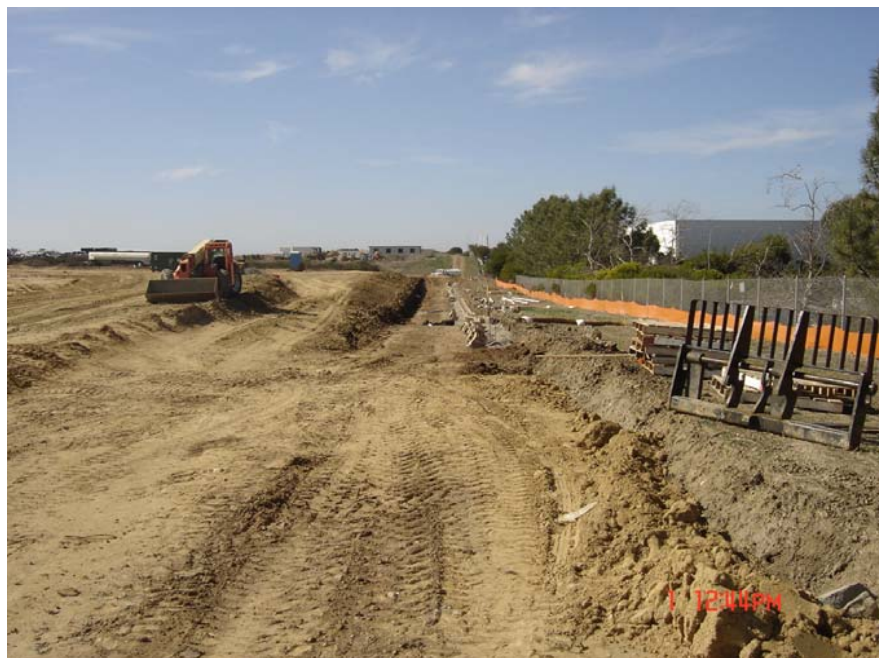
Station 6, February 1, 2006. Looking West.
