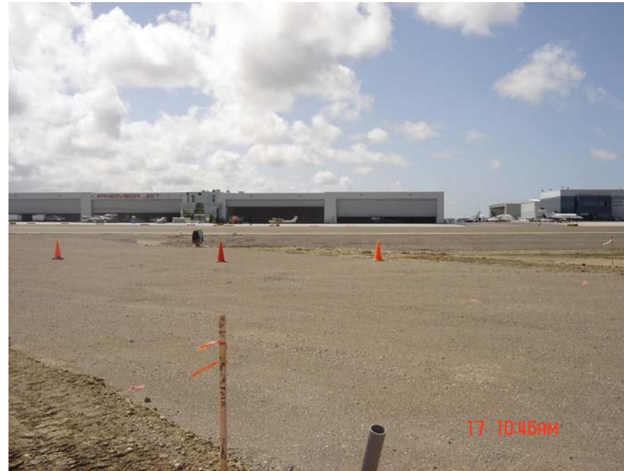
Station 2, April 17, 2006. Looking South.
