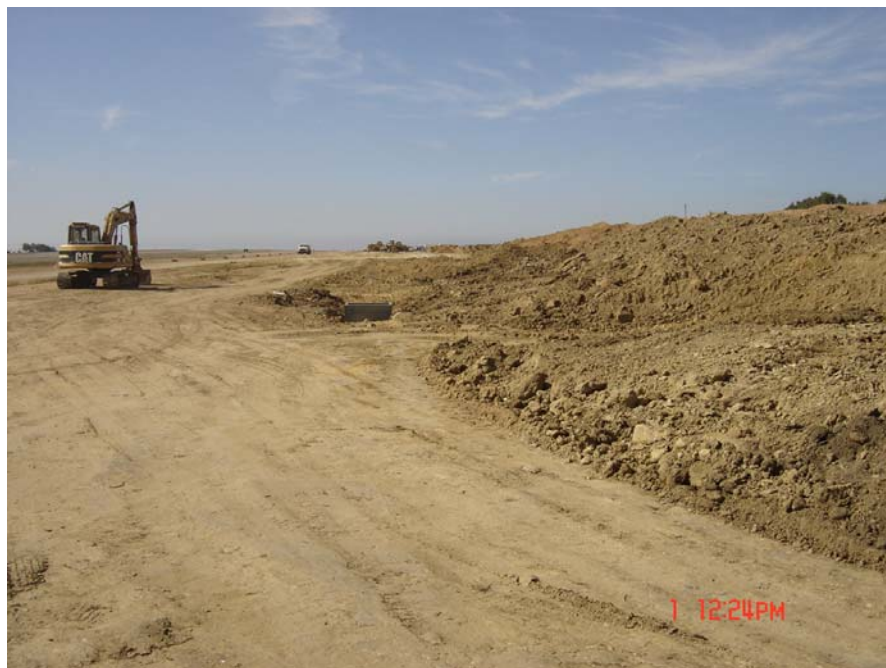
Station 2, February 1, 2006. Looking West.
