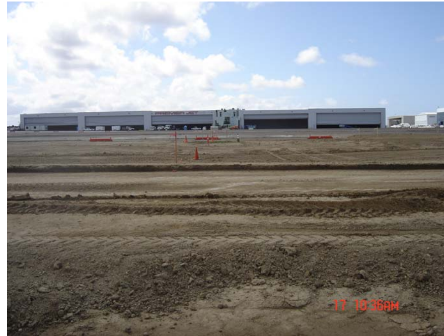
Station 1, April 17, 2006. Looking South
