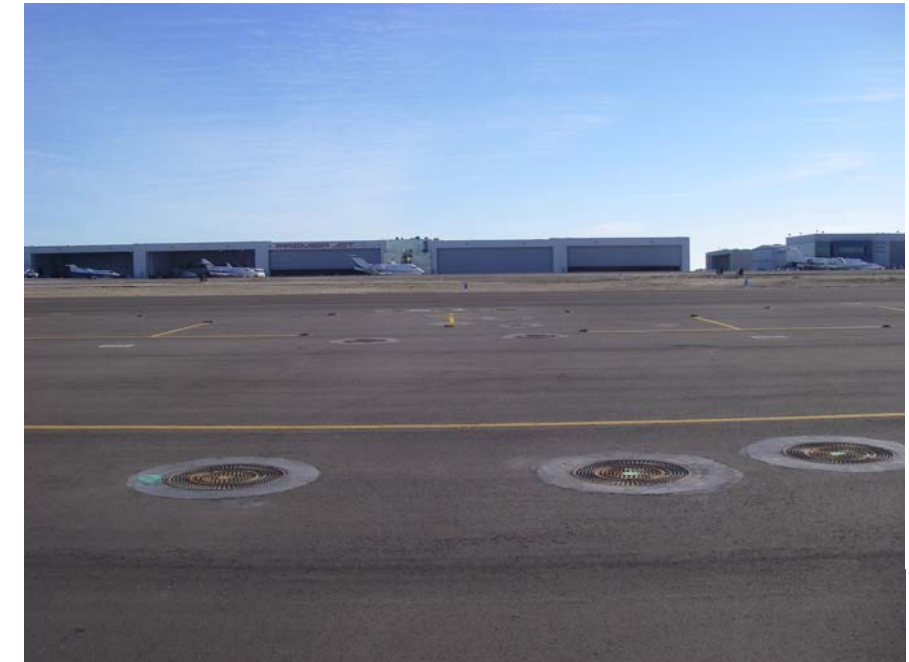
Station 4, January 3, 2007. Looking South
