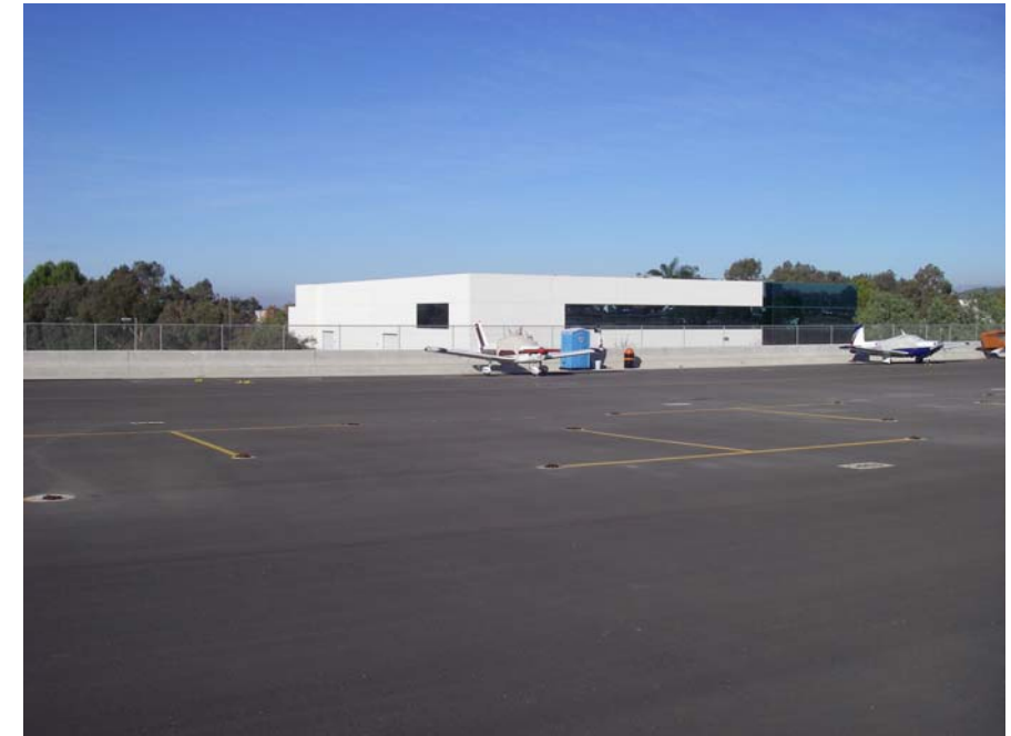
Station 2, January 3, 2007. Looking North
