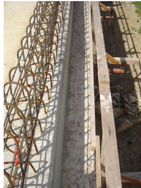
Station 4, April 17, 2006. Looking North.
