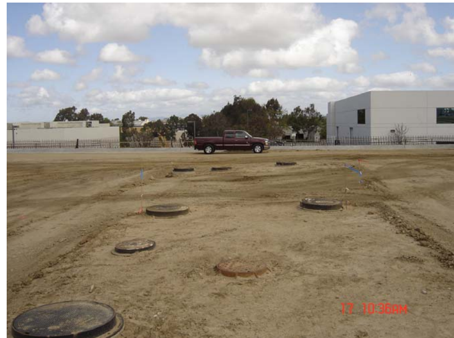
Station 1, April 17, 2006. Looking North
