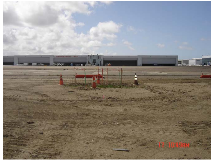
Station 3, April 17, 2006. Looking South.
