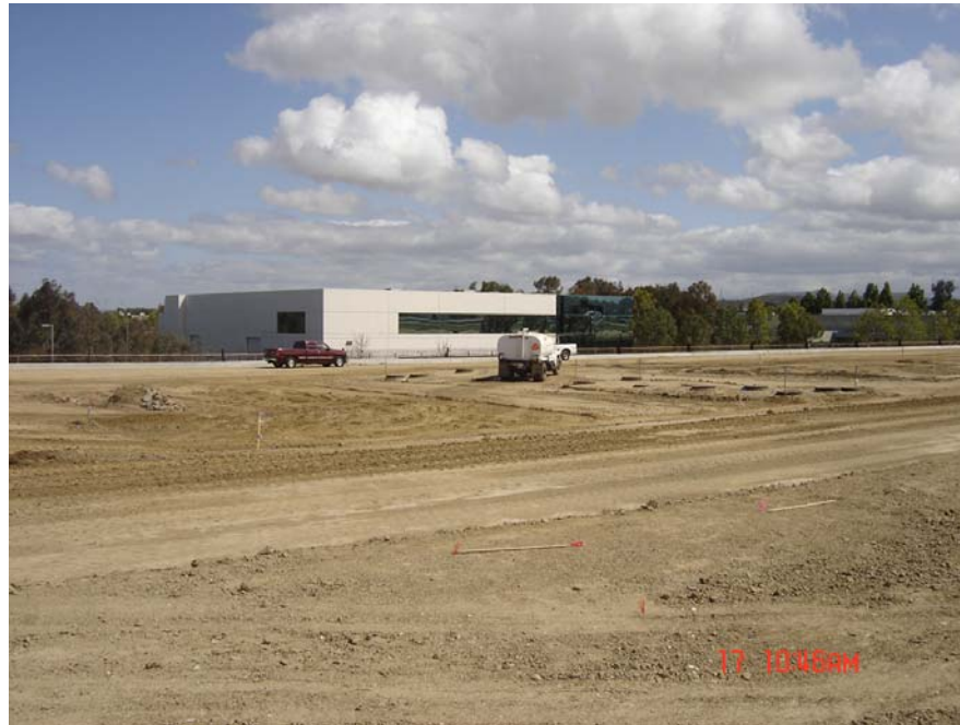
Station 2, April 17, 2006. Looking North.
