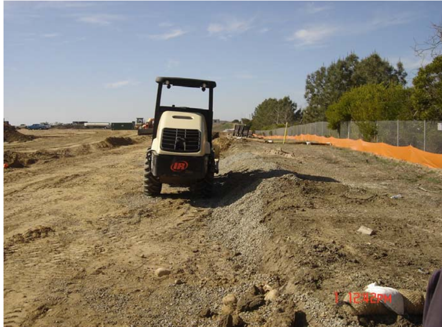
Station 5, February 1, 2006. Looking West.
