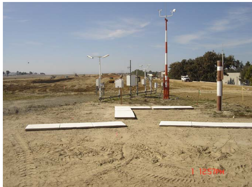
Station 7, February 1, 2006. Looking West.
