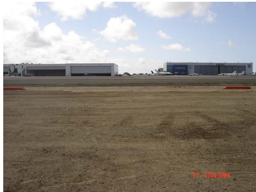
Station 6, April 17, 2006. Looking South.
