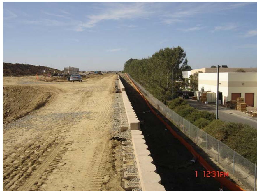
Station 4, February 1, 2006. Looking West.
