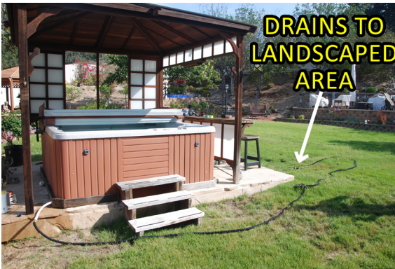
Spa water being drained to a landscaped area.
