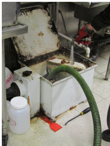
Cleaning a restaurant grease trap.
