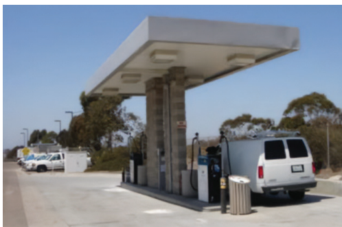
A covered fueling station is kept clean
