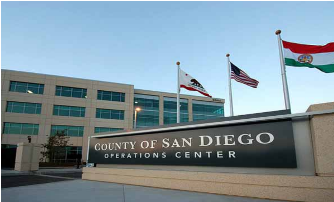
County Operations Center (COC)
