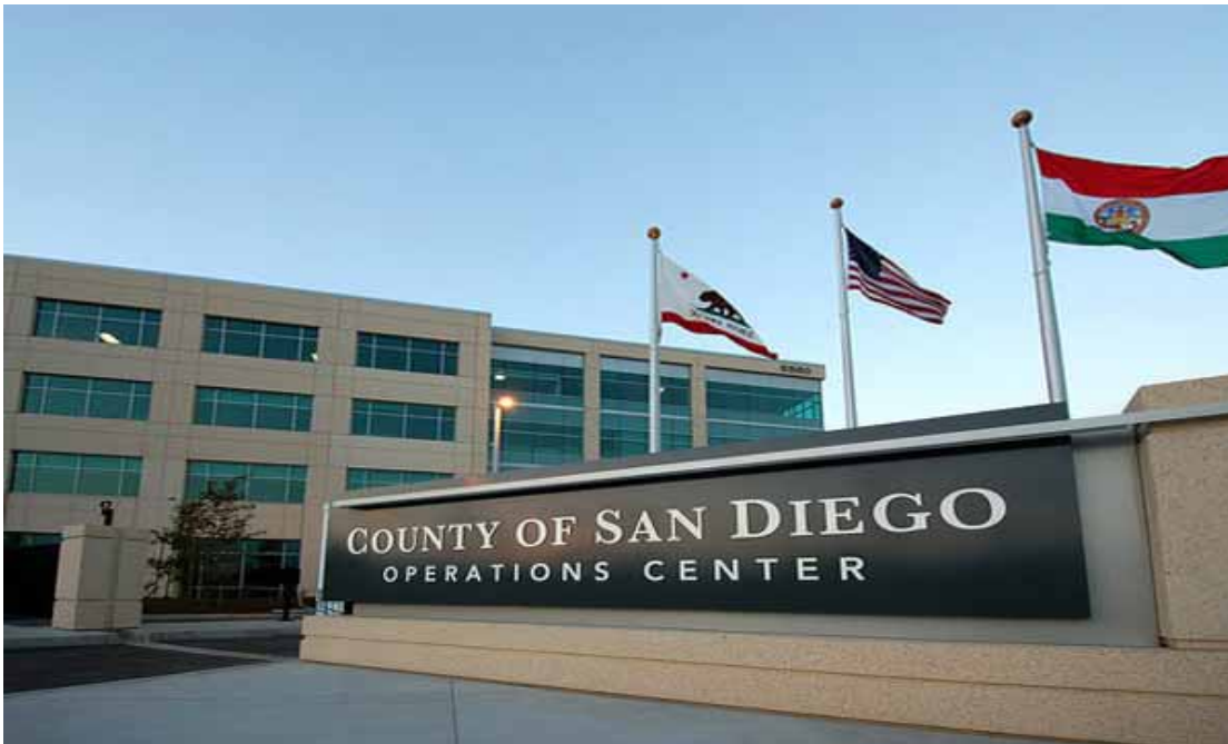
County Operations Center (COC)
