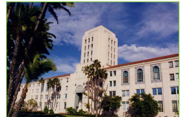
The red tile roof was replaced in 1998.
