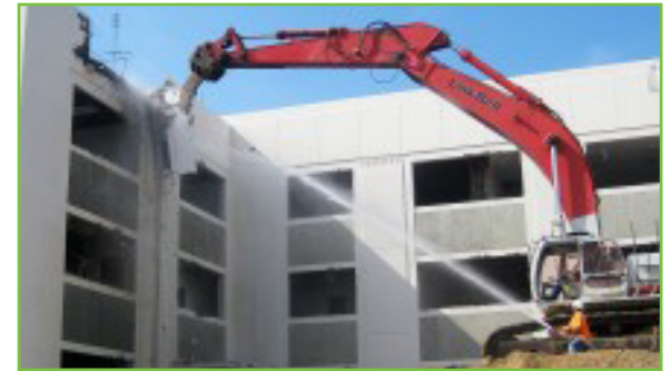
Demolition of the J.B. Askew building was completed in 2011.
