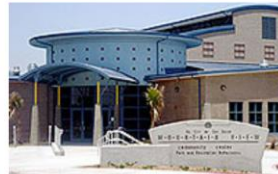
The Mountain View Community Center will serve as a temporary shelter for storm-impacted residents due to flooding in the Southeastern community. Photo: City of San Diego
