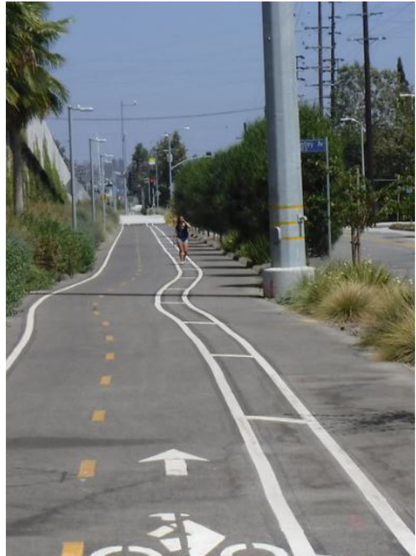
Example of a shared-use path in Los Angeles, California.
