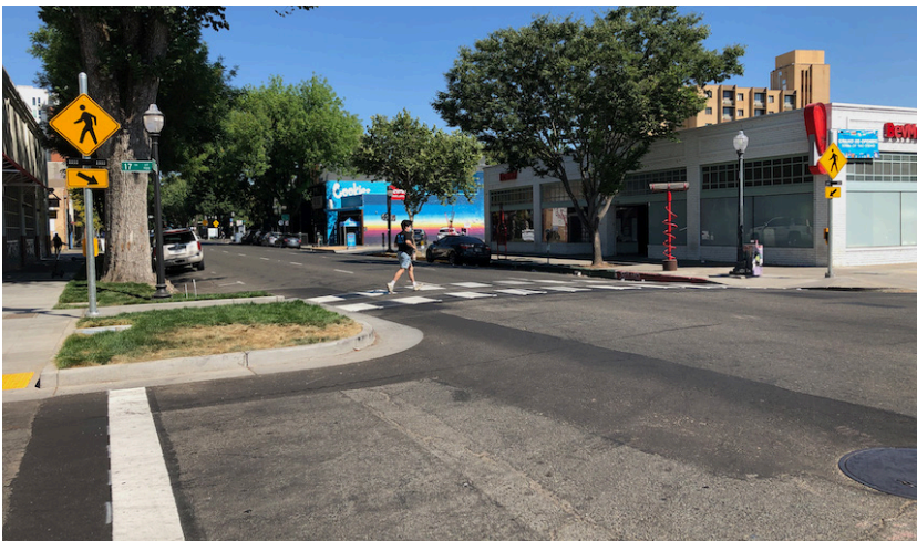
A crossing featuring RRFBs and curb extensions, Sacramento, CA.
