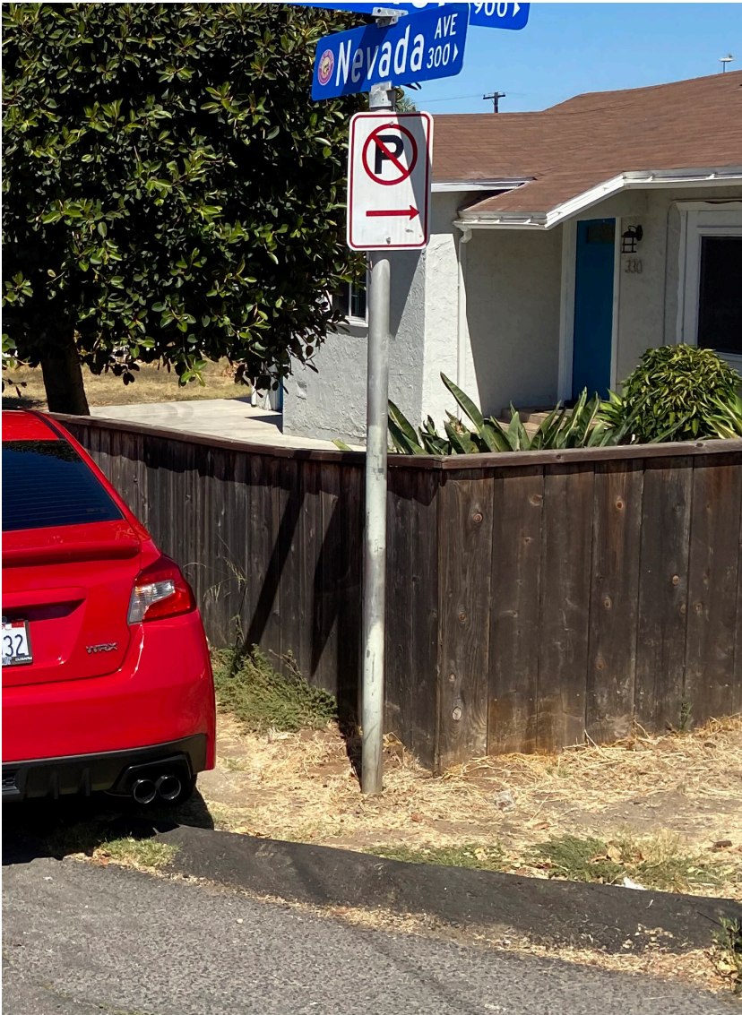
Some curbs in Townsite have no curb ramps.
