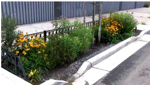
Photo 13: Bioswale incorporated into parkway to capture stormwater from the roadway. The dip in the curb allows the water to flow into the landscaped areas where the water then naturally filters through the soil and into the ground as opposed to flowing into storm drains.
