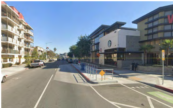
Photo 11: Example of bus stop along separated bikeway. (Long Beach, California)
