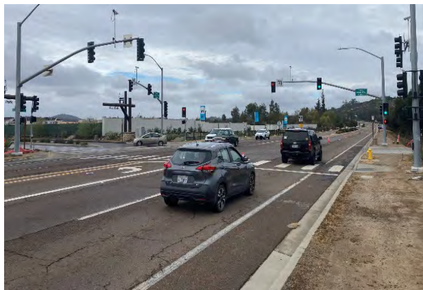
Photo 4: Traffic signal constructed in 2021 at the intersection of Valley Center Road and Park Circle Way as part of the Park Circle development
