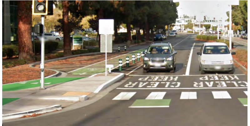
Photo 9: Example of bicycle lane ramping up to sidewalk level at curb extension (Fremont, California).
