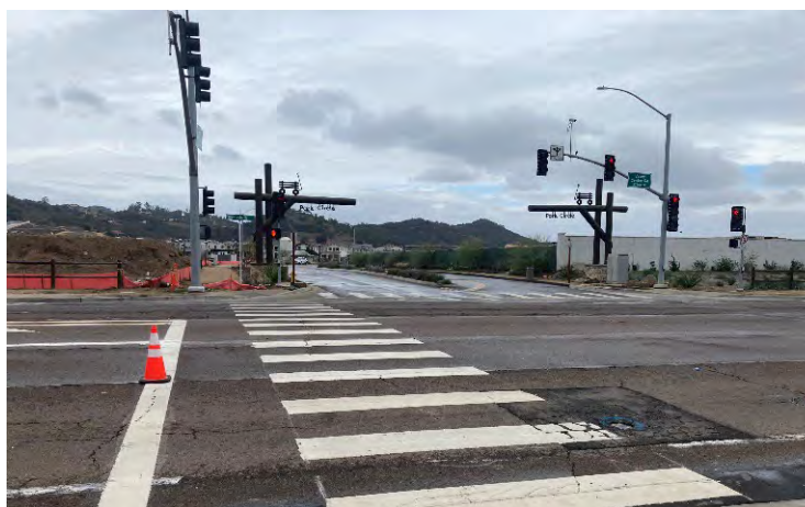
Photo 7: Continental crosswalk marking at Mirar de Valle Road along Valley Center Road.
