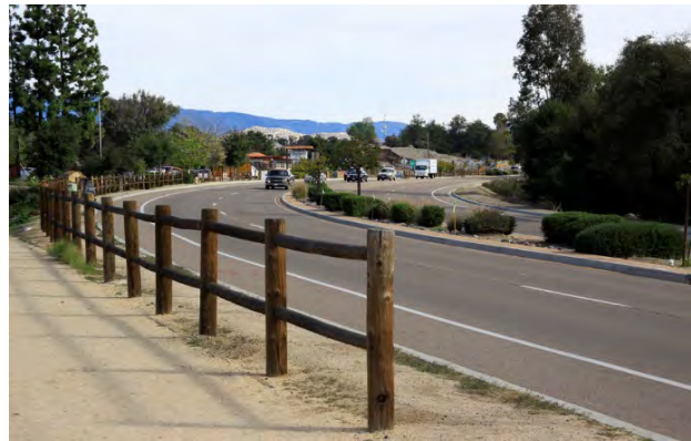
Photo 1: Valley Center Road currently has four travel lanes, a mix of raised and striped medians, the Heritage Trail, Class II bike lanes, and intermittent sidewalks.
