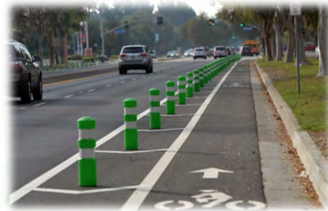
Figure 24: Class IV Bikeway with buffer and flexible delineator posts along Leucadia Boulevard looking westbound
