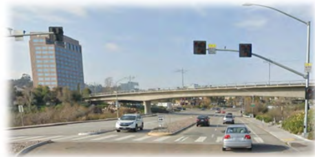
Figure 14: HAWK signal on Mission Center Road in Mission Valley
