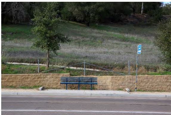
Figure 12: Typical Bus Stops with Bench and Sign
