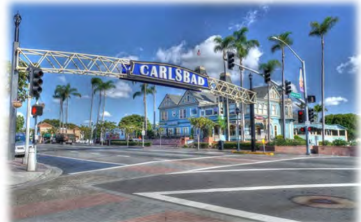
Figure 27: City of Carlsbad Gateway Feature
