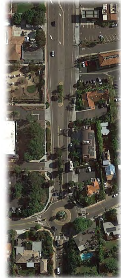
Figure 9: Single-lane Roundabout with taper at Santa Fe Drive & Devonshire Drive in Encinitas
