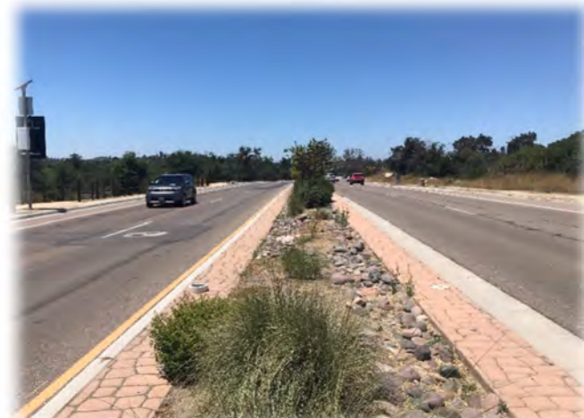
Figure 17: Raised Landscaped Median on Valley Center Road west of Cole Grade Road
