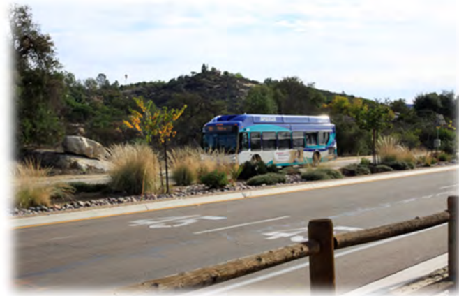
Figure 16: Raised Landscaped Median on Valley Center Road west of Lilac Road
