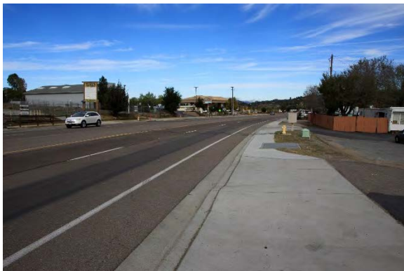
Figure 1: Looking northbound near Woods Valley Road
