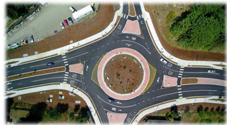
Figure 8: Two-Lane Roundabout at Tremont Street & Pottery Avenue in Washington
