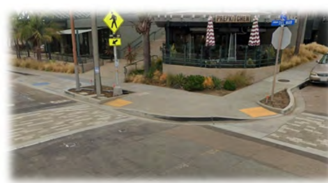
Figure 12: Curb extensions at Camino Del Mar & 12 th Street in Del Mar
