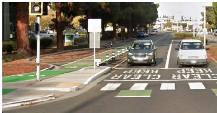
Photo 7: Example of bicycle lane ramping up to sidewalk level at curb extension (Fremont, California)
