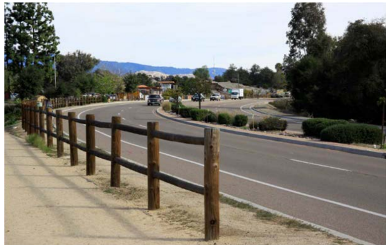
Photo 1: Valley Center Road currently has four travel lanes, a mix of raised and striped medians, the Heritage Trail, Class II bike lanes, and intermittent sidewalks.
