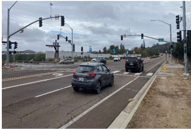
Photo 5: Traffic signal constructed in 2021 at the intersection of Valley Center Road and Park Circle Way as part of the Park Circle development project
