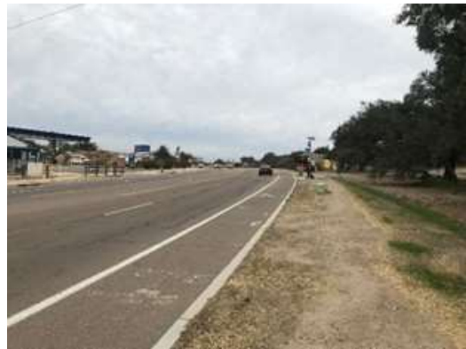
Photo 10: Example of existing gap in sidewalk on south side of Valley Center Road in the North Village
