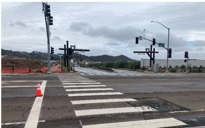
Photo 11: Continental crosswalk marking at the Valley Center Road / Park Circle Way intersection
