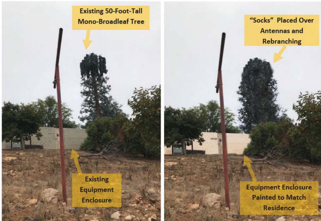
Figure 1: View on site of existing (left) and proposed (right) mono-broadleaf tree and equipment enclosure, looking northwest.
