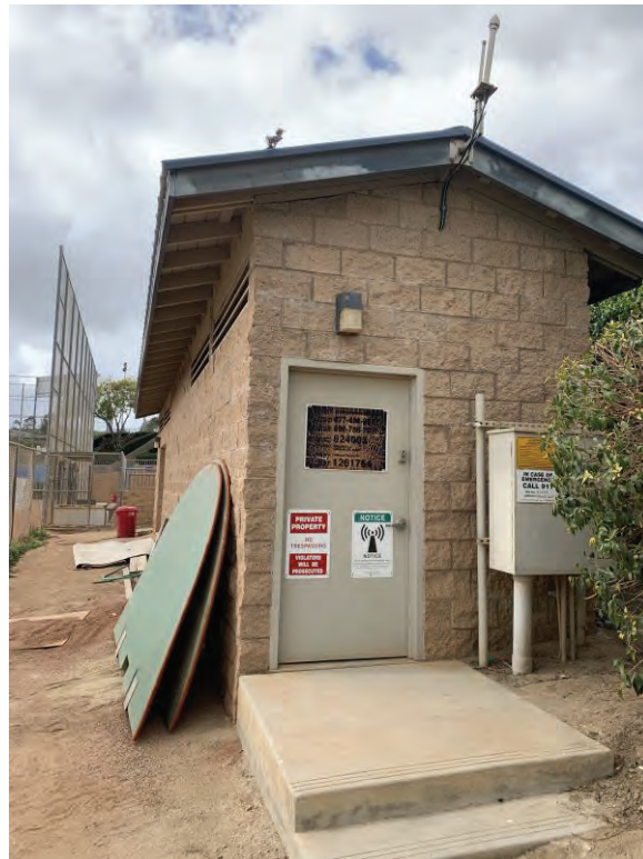
View north of existing equipment shelter from ballfield
