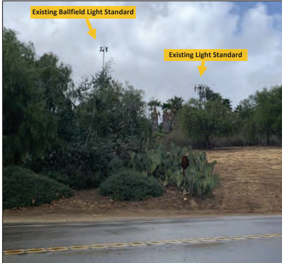
Figure 2: View of existing 75-foot-tall light standard, looking north from Olive Hill Road.
