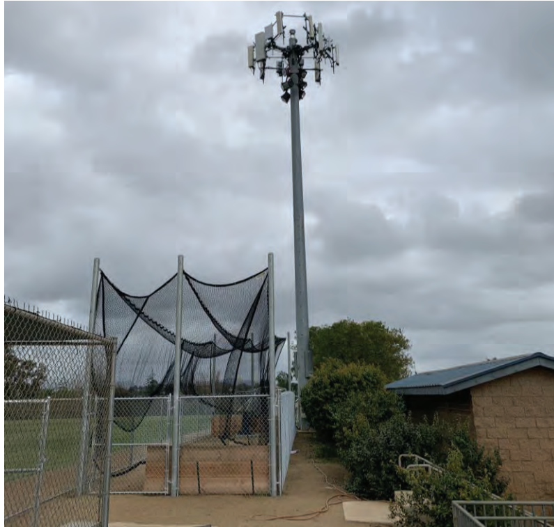
View south on ballfields of existing light pole with antennas
