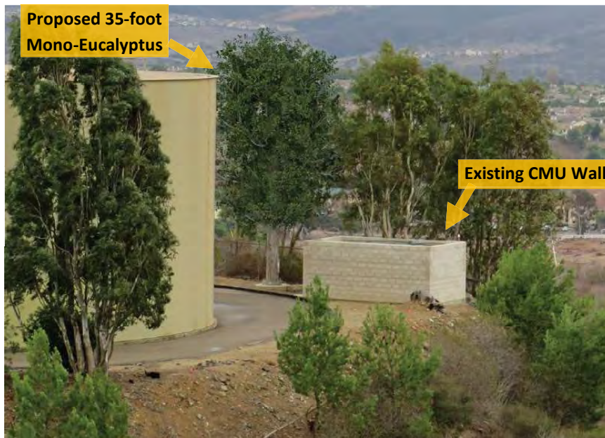
Figure 2: View of proposed 35-foot-tall mono-eucalyptus and 8-foot-tall CMU wall, looking south on project site.
