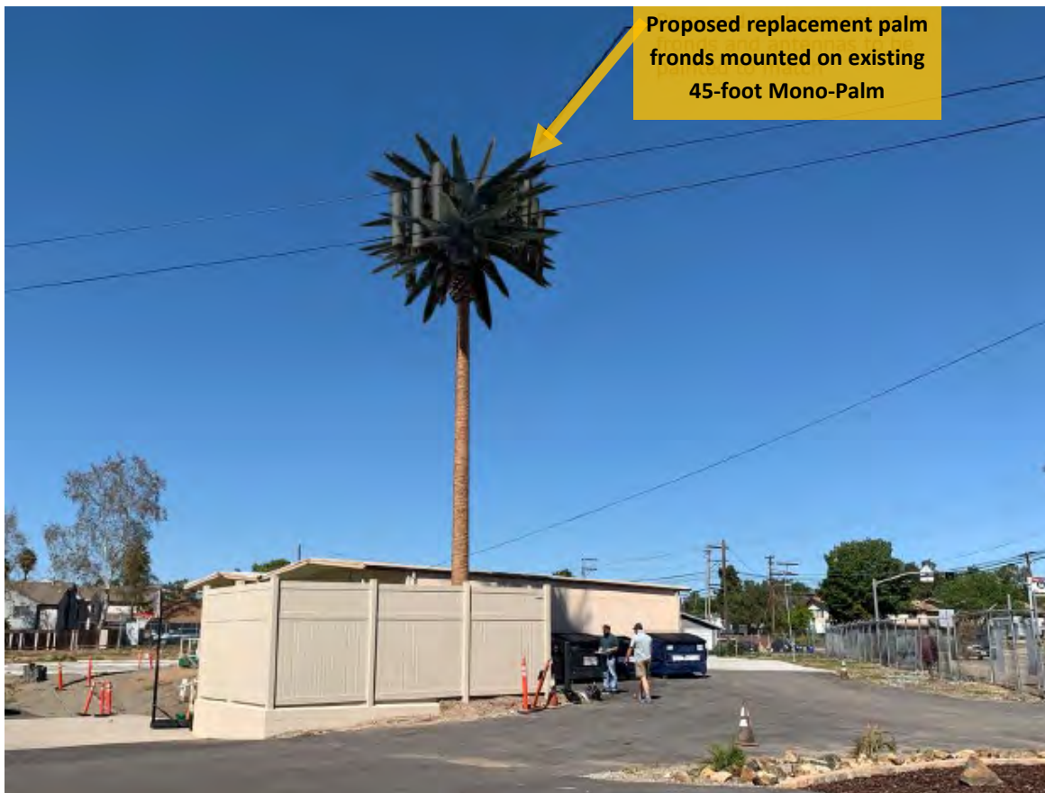
Figure 2: View of existing 45-foot-tall mono-palm with proposed additional palm fronds, looking north onsite.
