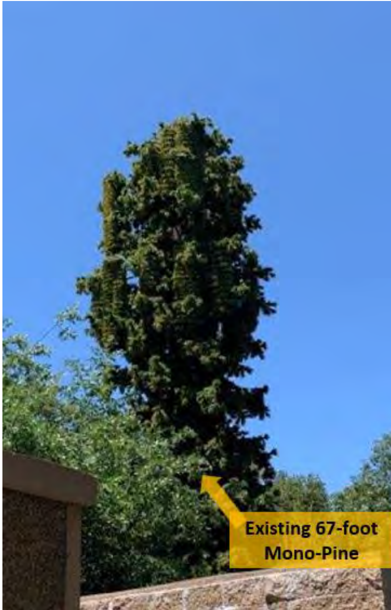
Figure 1: View of the existing mono-pine tree, looking south on project site.
