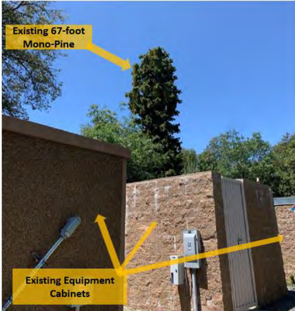
Figure 2: View of existing 67-foot-tall mono-pine and equipment shelters looking south on project site.
