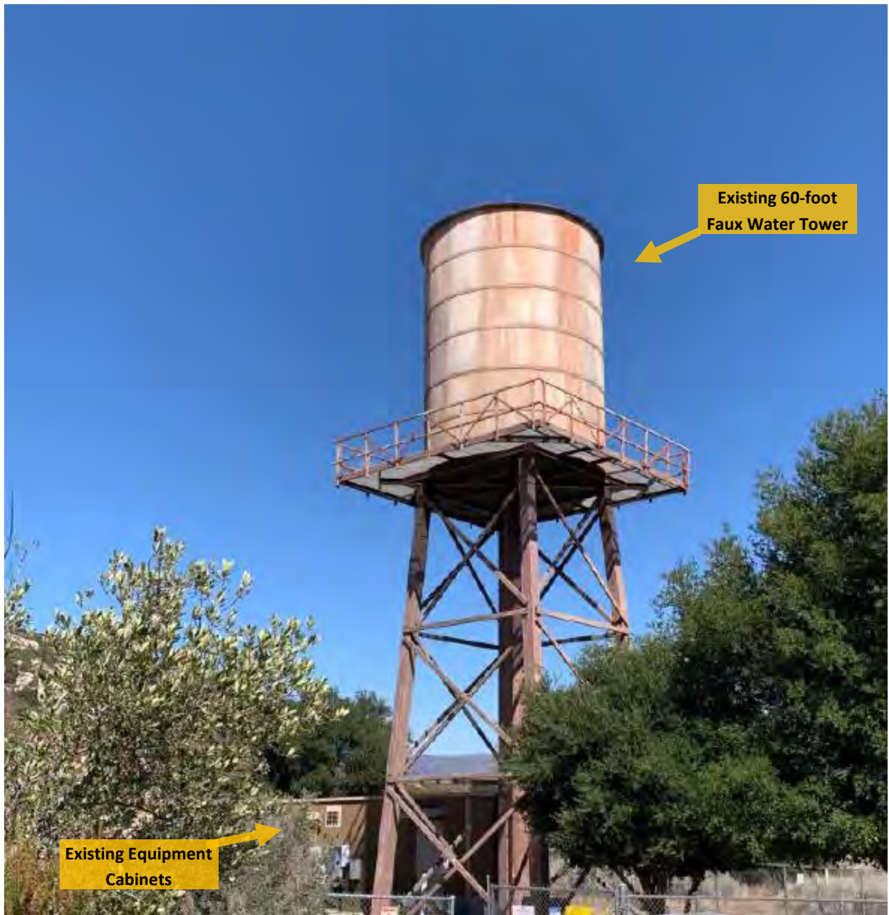
Figure 1: View of the existing faux water tower and equipment cabinets, looking north on project site.
