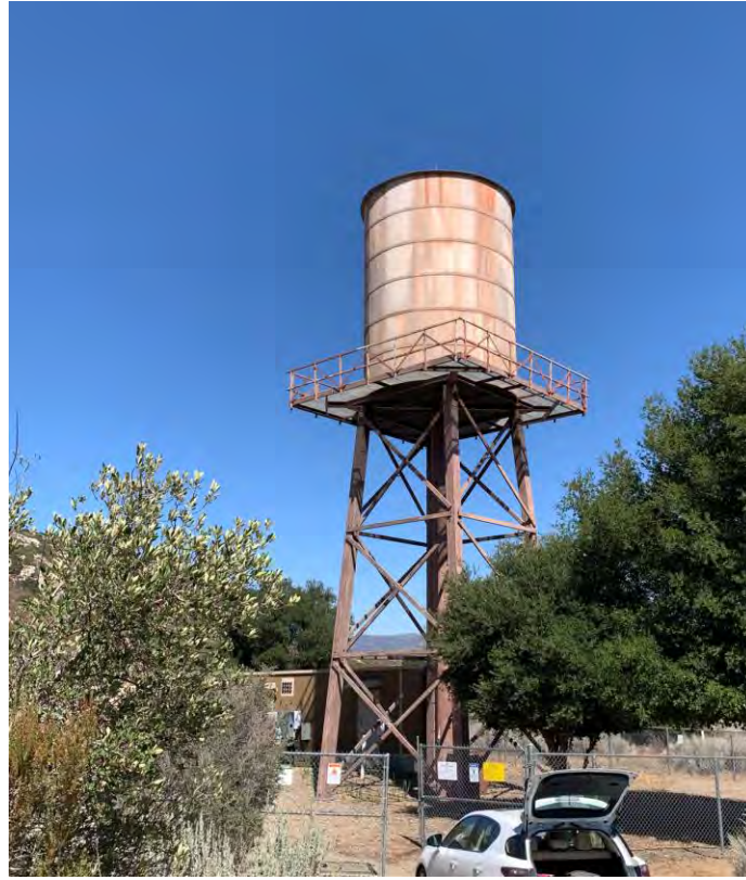
View north of water tank from entrance to compound
