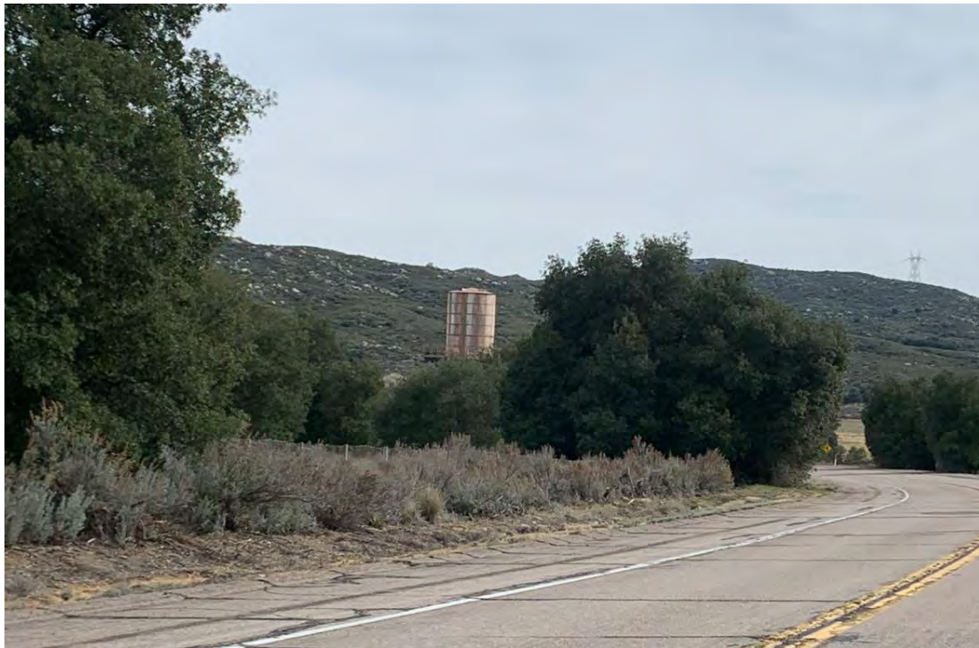
View northeast of site from Old Highway 80
