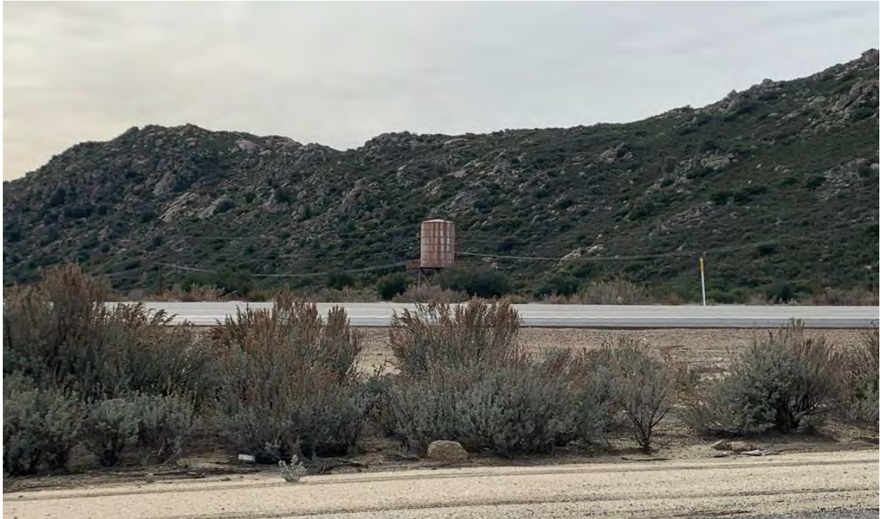
View south toward site from westbound Highway onramp
