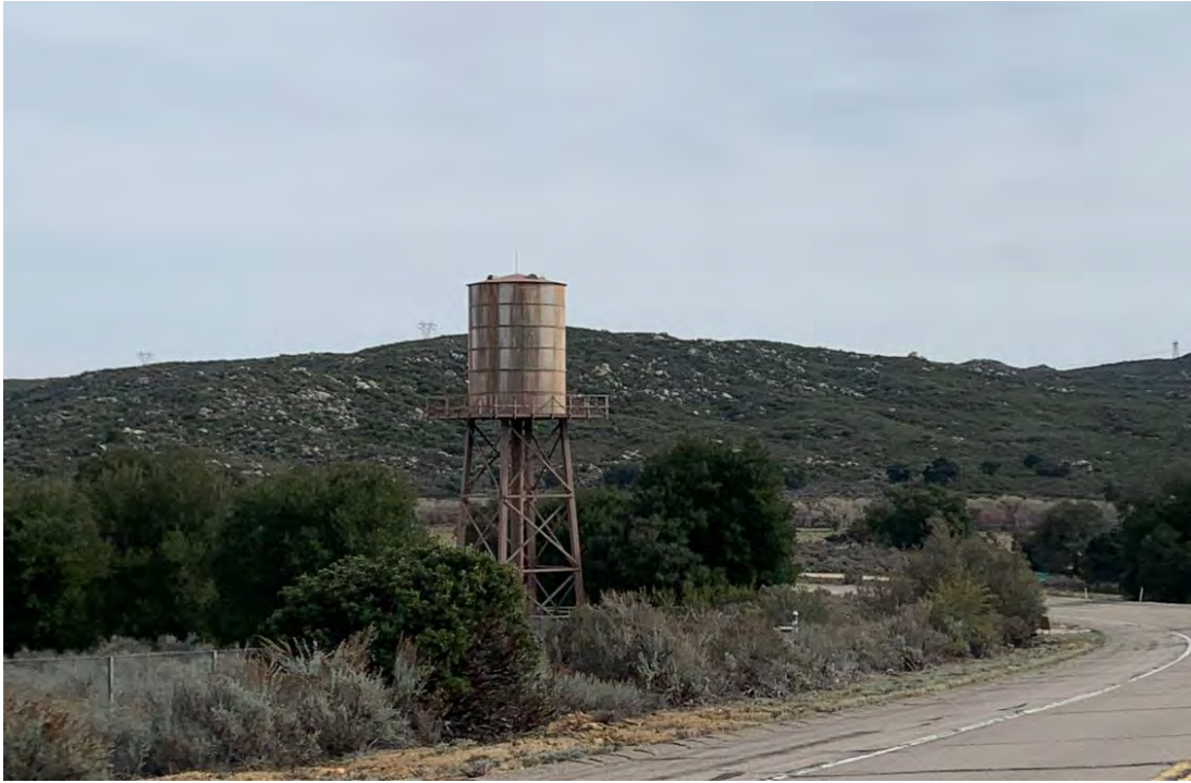
View northeast of site from Old Highway 80
