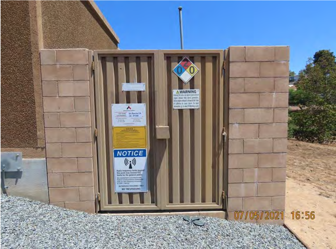
Existing equipment area
