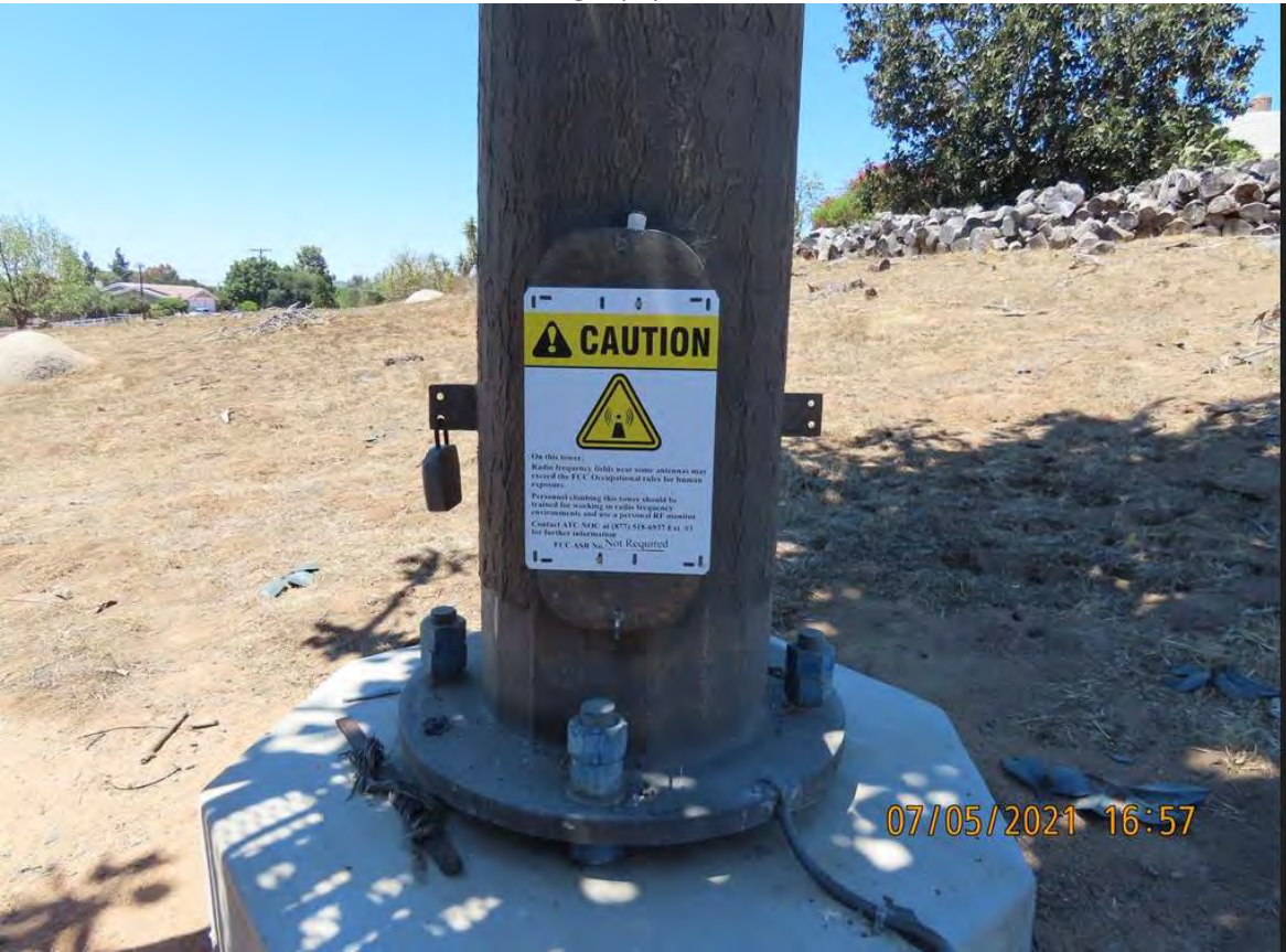
View of base of pole
