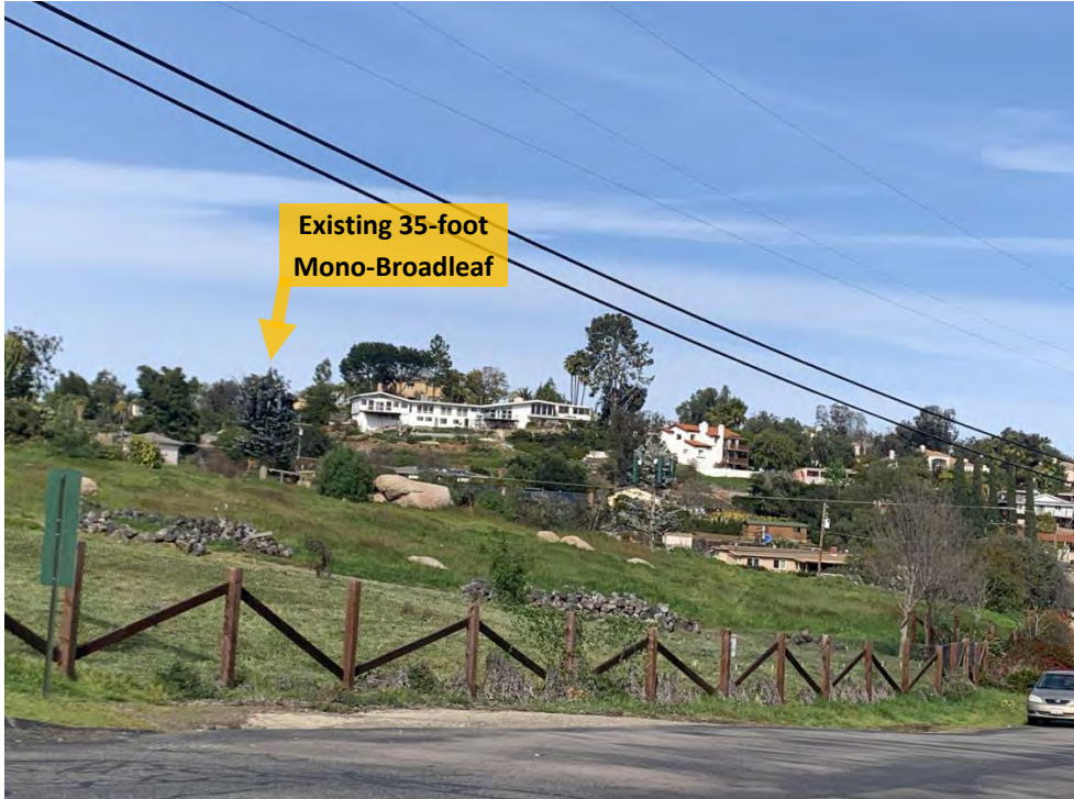
Figure 3: View of project site looking Northwest towards facility from Purer Rd.
