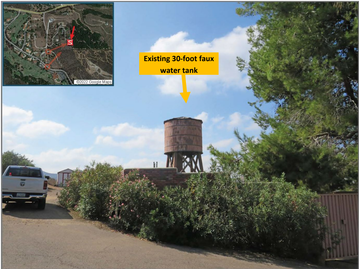
Figure 1: View of existing 30-foot-tall faux water tank looking southwest from the onsite access road.
