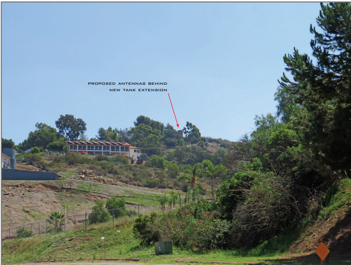
LOOKING SOUTHEAST FROM GOPHER CANYON ROAD
