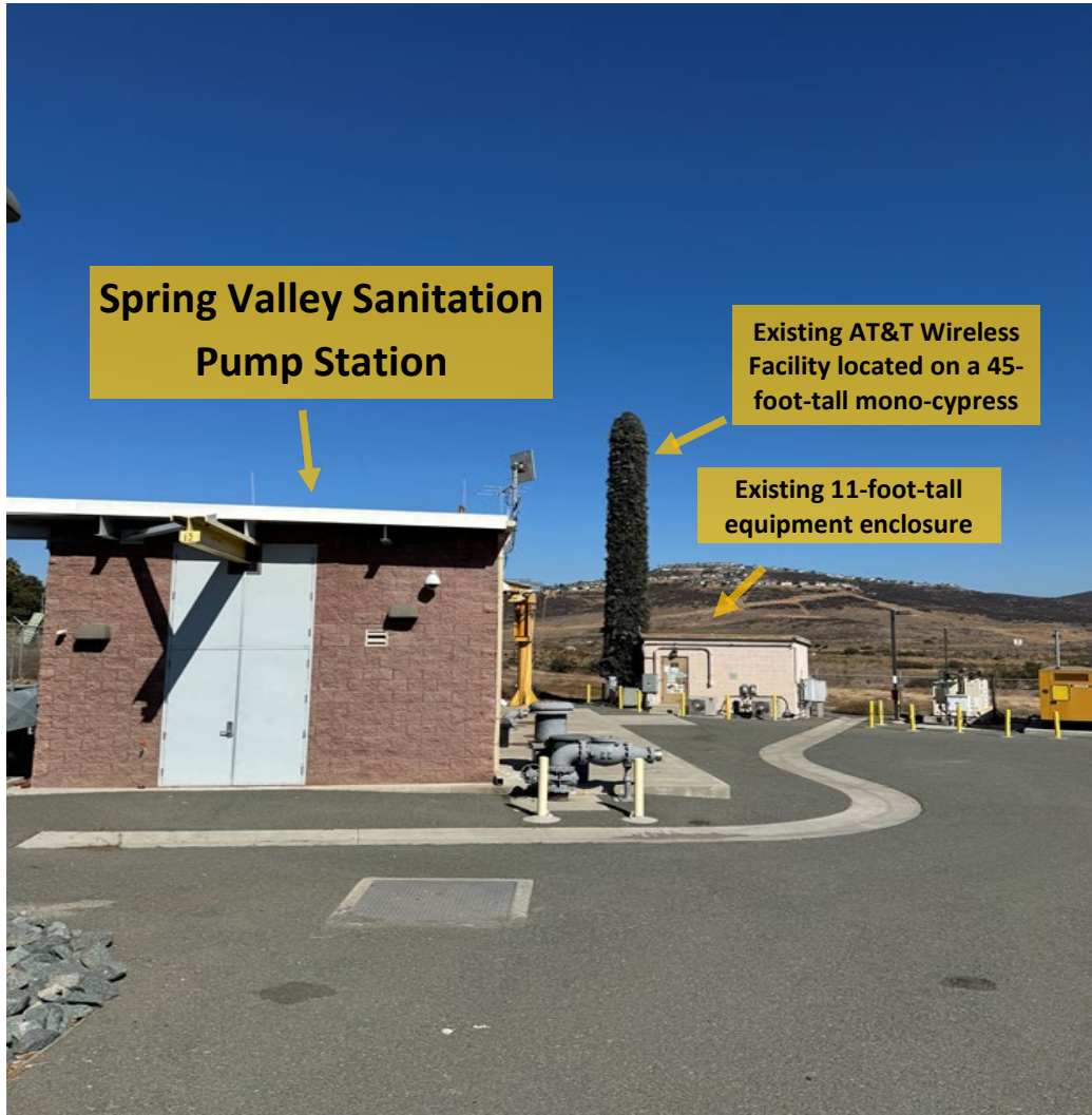
Figure 2: (Left) Existing Spring Valley Pump Station (Center) Existing AT&T 45-foot-tall wireless facility, (Right) Existing CMU equipment enclosure.
