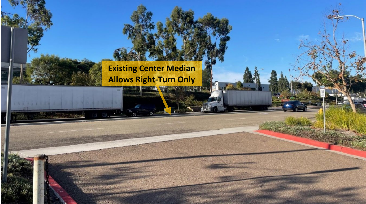
Figure 9: Existing Project Access and Driveway (Looking South)
