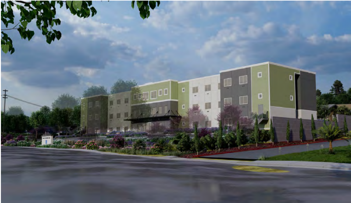
Figure 5: Looking Southeast at Building 4 across Bradley Avenue
