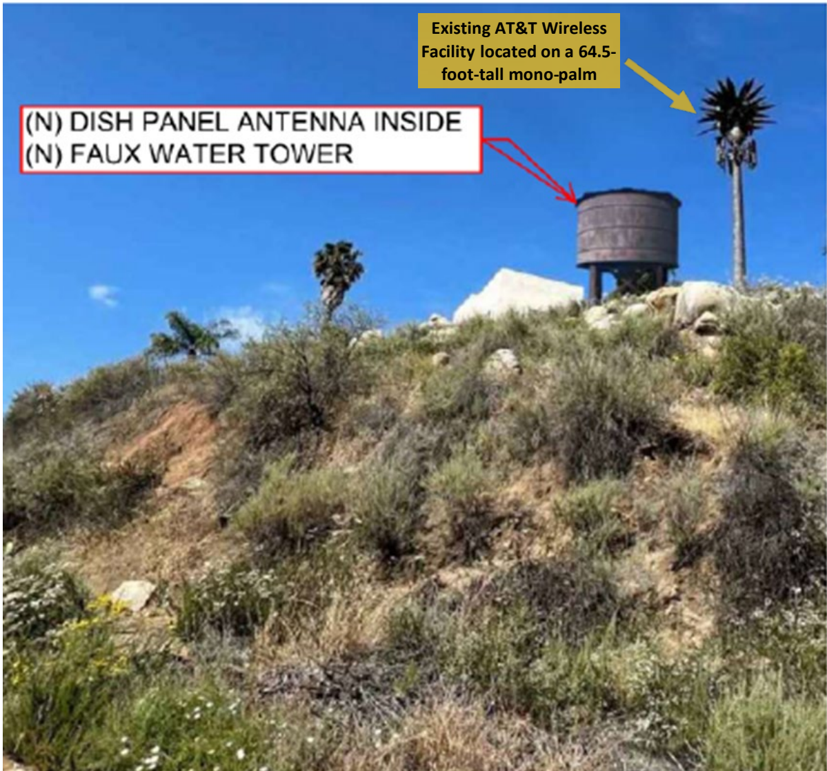
Figure 1: (Left) Proposed Dish 17.6-foot-tall faux water tower wireless facility. (Right) Existing AT&T 64.5-foot-tall mono-palm wireless facility.
