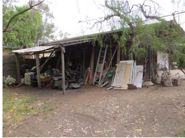
Photograph 15: Storage area on west side of garage.
