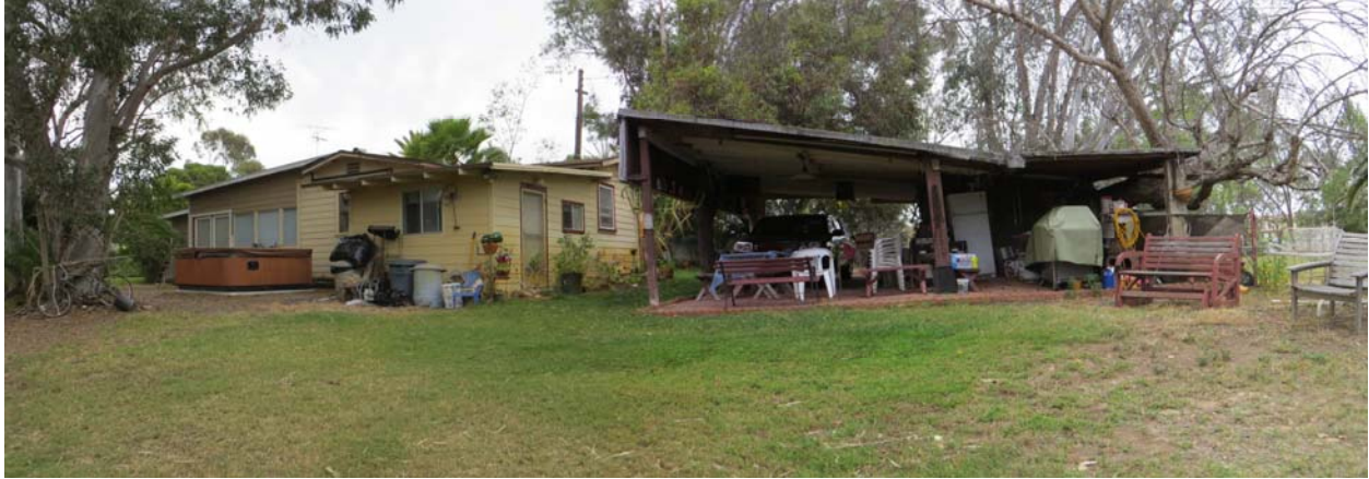
Photograph 9: Southeast view of the caretaker's cottage and the carport. Just out of view on the right side of this photograph is the water tank shown in Photograph 17.
