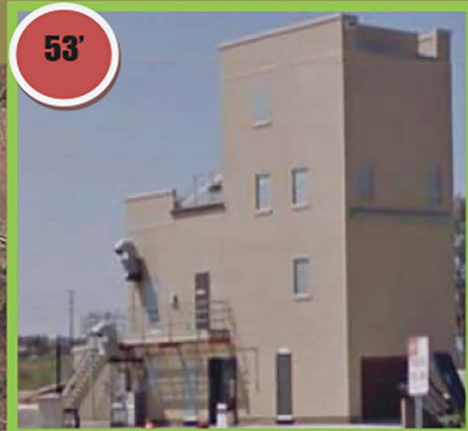
53' Fire Station tower 53' 200' W
