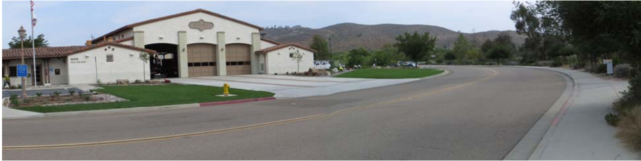
Photograph 2: Northwest view of Four Gee Road and west adjoining fire station.
