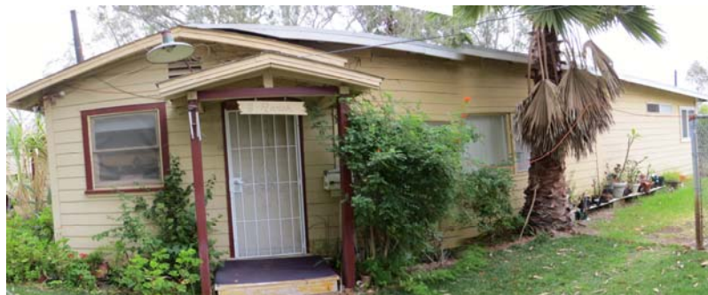
Photograph 8: South view of the caretaker's cottage.
