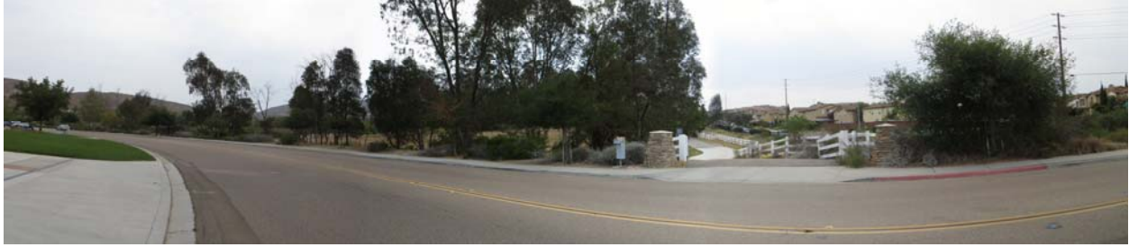
Photograph 1: East-northeast view of the west Property parcel and entrance to the main Property parcel with Four Gee Road in the foreground. In the back right of the photograph is the La Viña tract.
