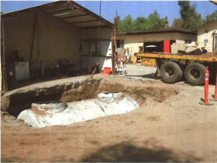
SITE LOOKING EAST
