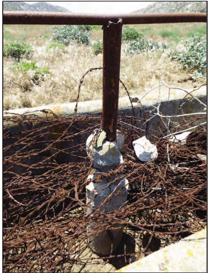
b. Close-up of Concrete Encased Trough Pipe, Looking West (PR-05430-048)
