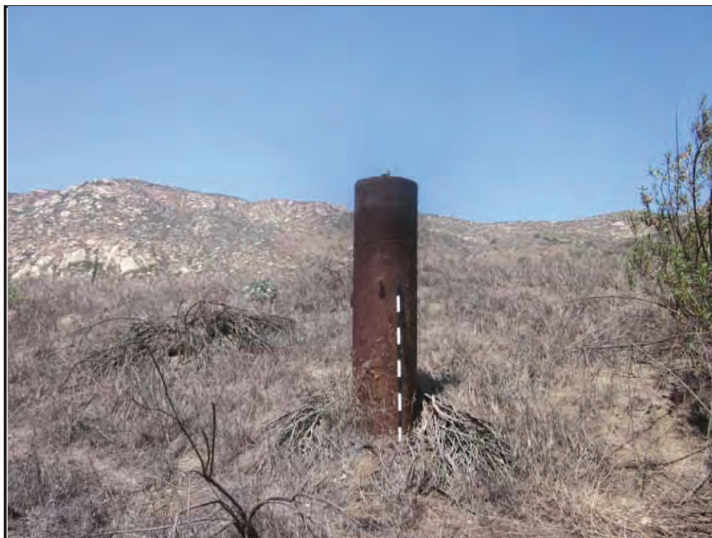
b. Overview of P-37-035818, Looking North
