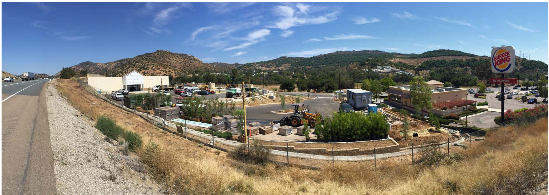
Figure 3-2. KOP 1 – Looking Southeast Towards Project Site from Eastbound I-8
