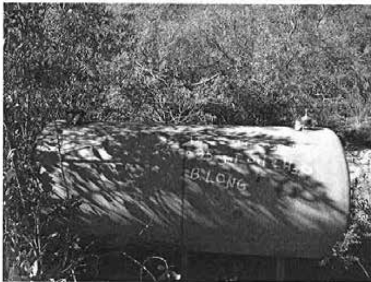
Tank was uprighted and the openings were secured
