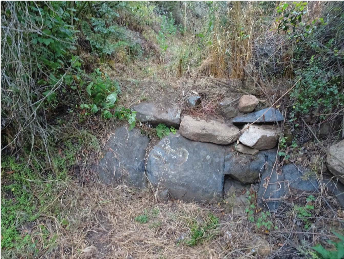
Figure 3. Upper Rock Drop Structure/Grade Control near Middle of Reach 1
