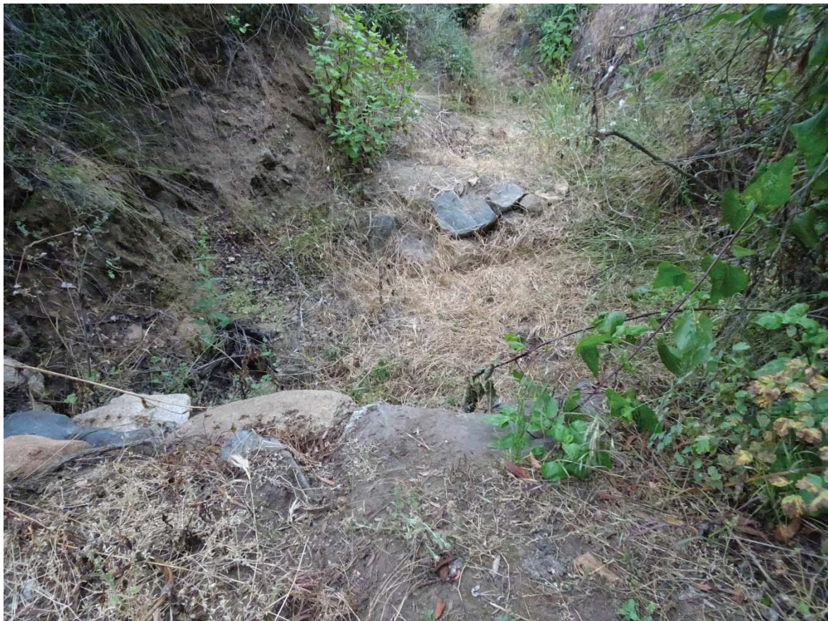
Figure 4. Looking Downstream towards Lower End of Reach 1
