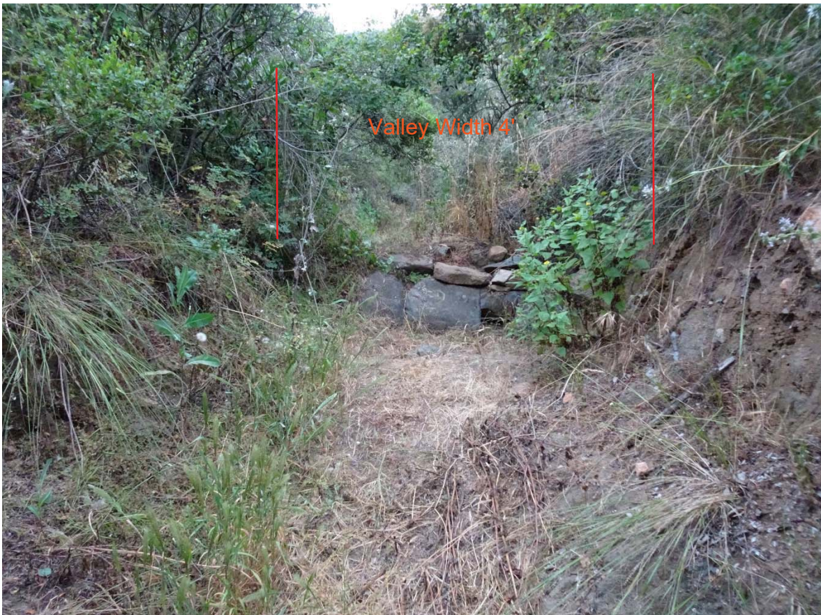
Figure 2. Looking Upstream from Middle of Reach 1 (towards upper rock grade control)
