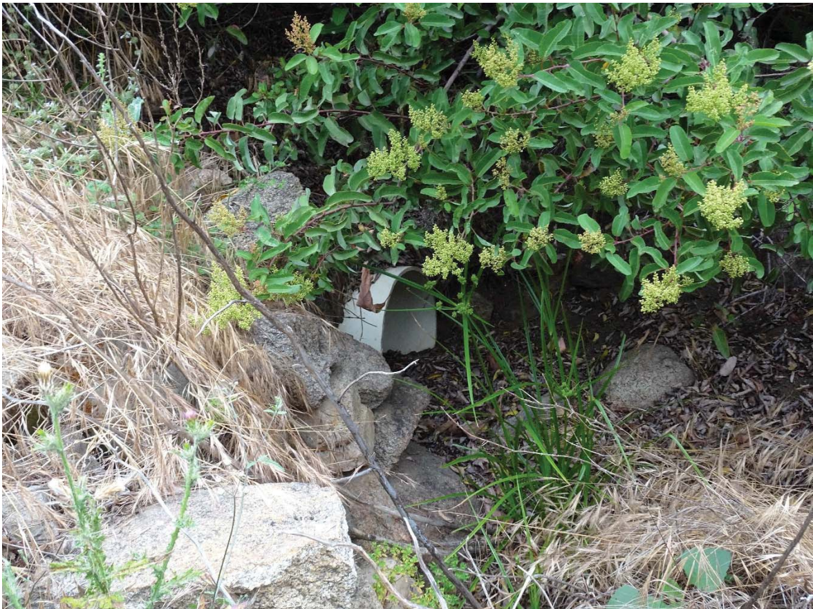
Figure 14. Roadway Culvert at Lower End of Reach 4
