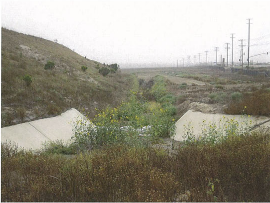
Figure 9. Looking Downstream at Reach 1 (POC 2) from 2011 Study
