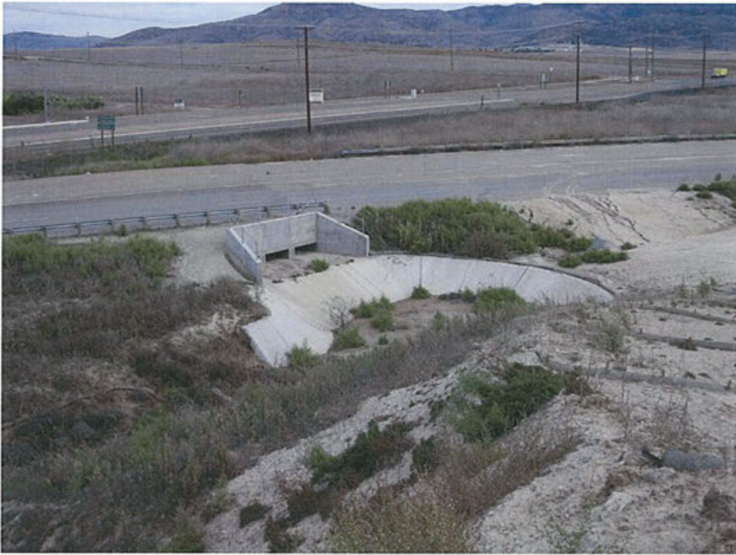
Figure 3. Box Culverts and Stilling Basin (Site is Behind Upper Road)
