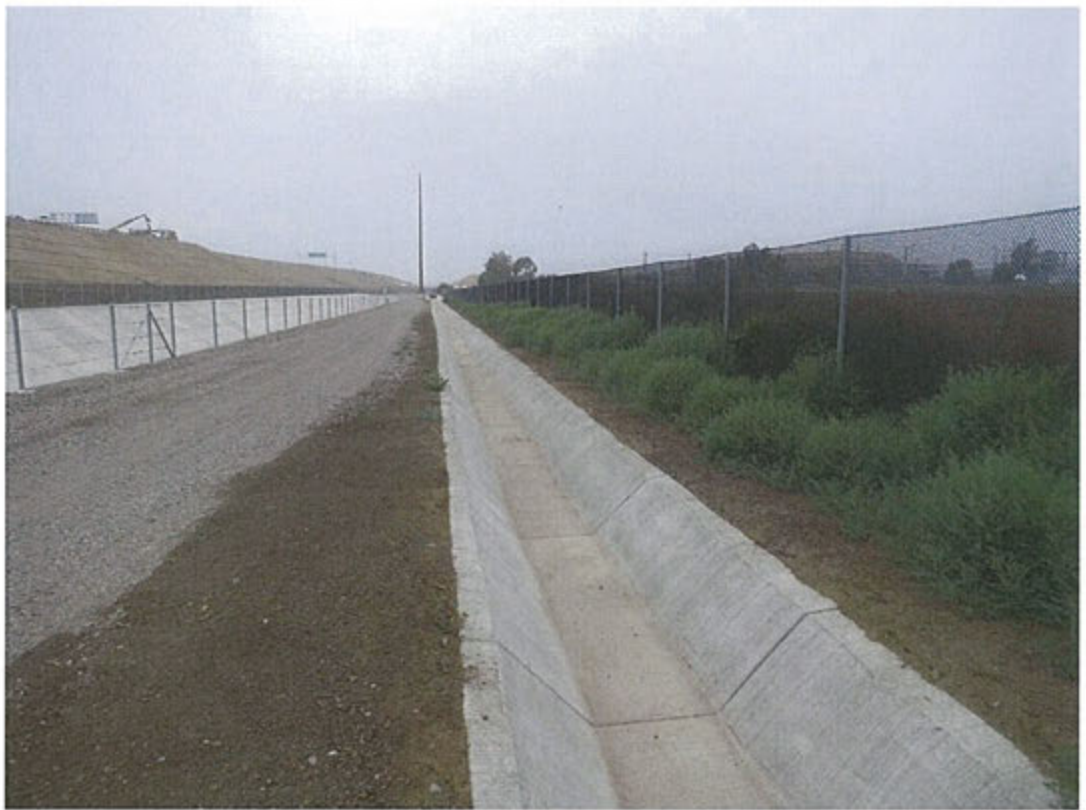
Figure 6. Caltrans Concrete Channel (Permanent Grade Control) at Lower End of Reach 2
