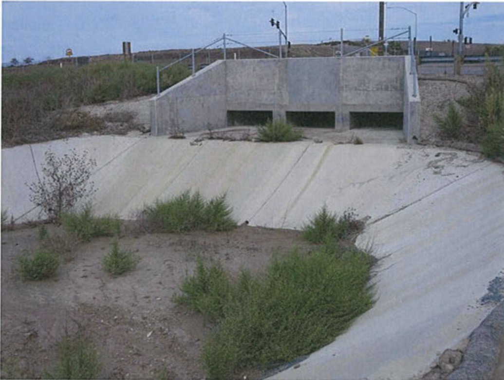
Figure 1. Box Culvert Outlets into Stilling Basin
