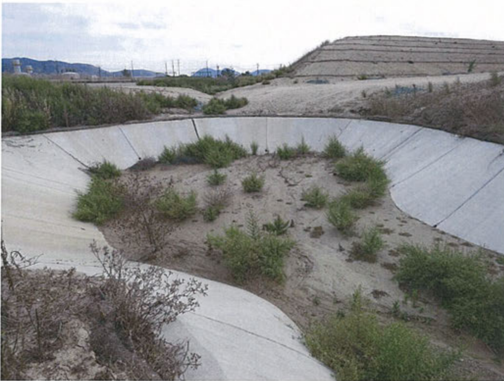
Figure 2. Stilling Basin (Box Culverts to Left of Photograph)
