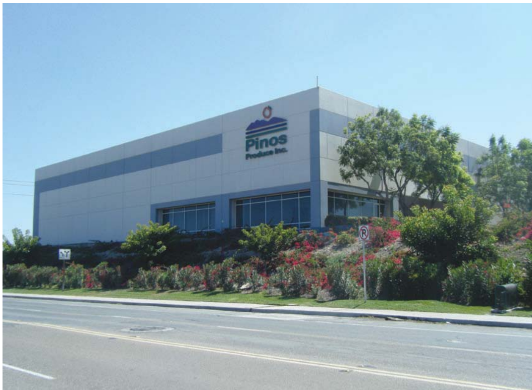
1) View of 1710 Dornoch Court, adjacent to the south of the Site.
