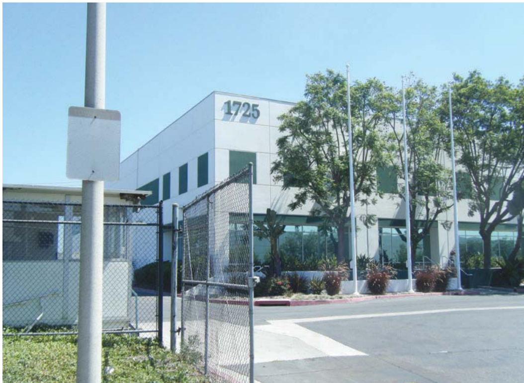
2) View of 1725 Dornoch Court, adjacent to the south of the Site.
