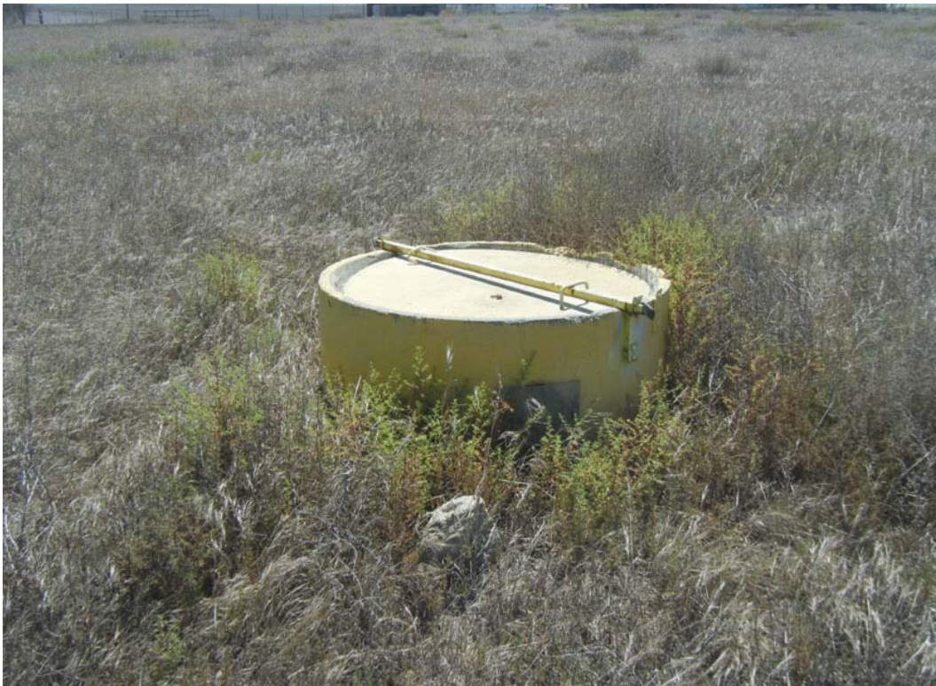
1) View of a water main at the southern central portion of the Site.
