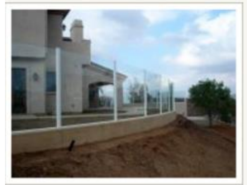
Example non-combustible fire wall
