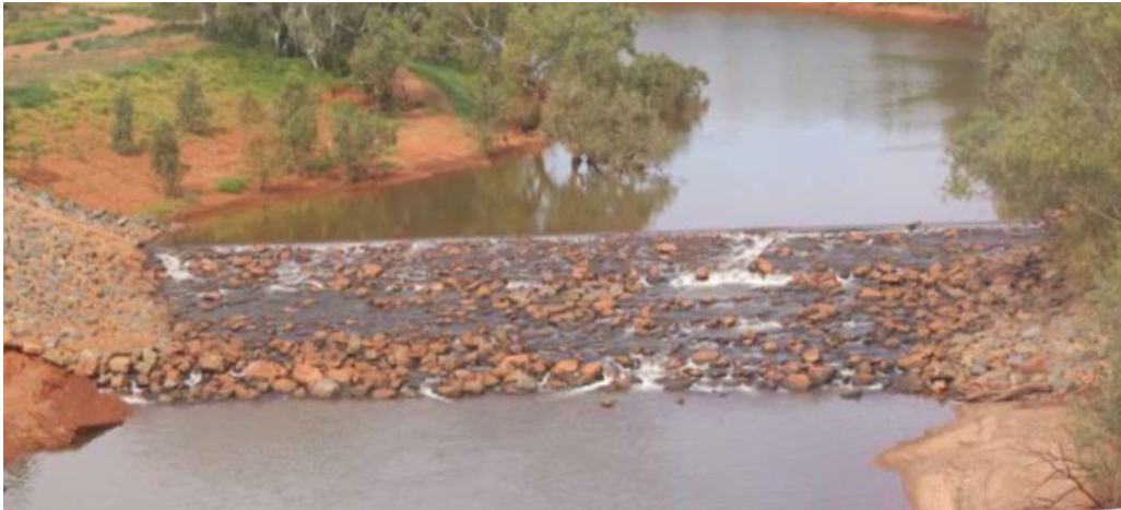
Figure A-1 Example of a Low-level Weir that Detains Streamflow in Northwestern Australia
