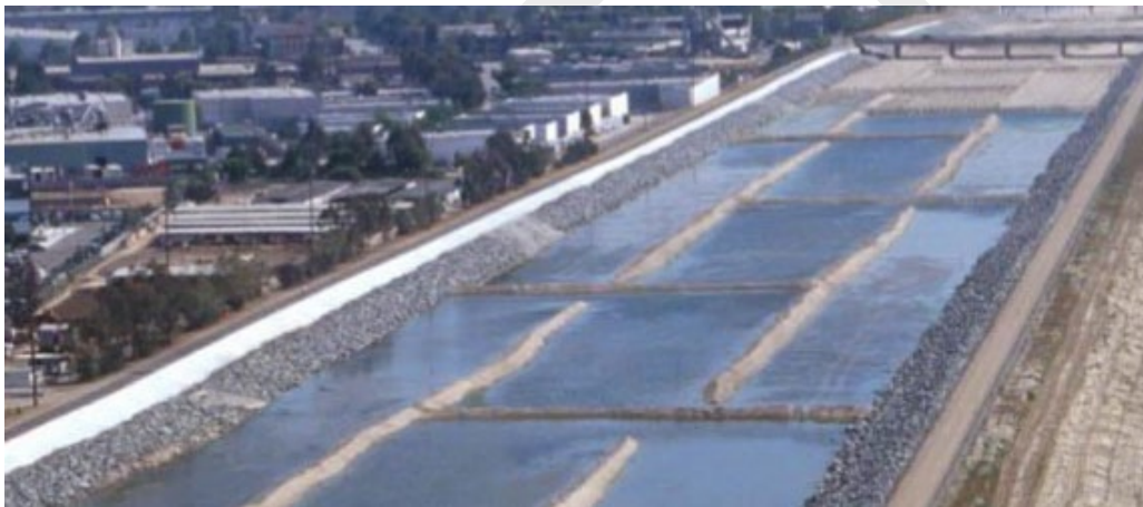
Figure A-2 Example of T and L Levees in Santa Ana River
