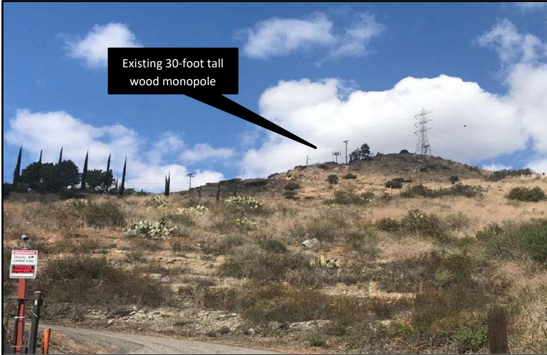
Figure 1(a): Existing 30-foot tall wooden monopole looking north from Hwy 76
