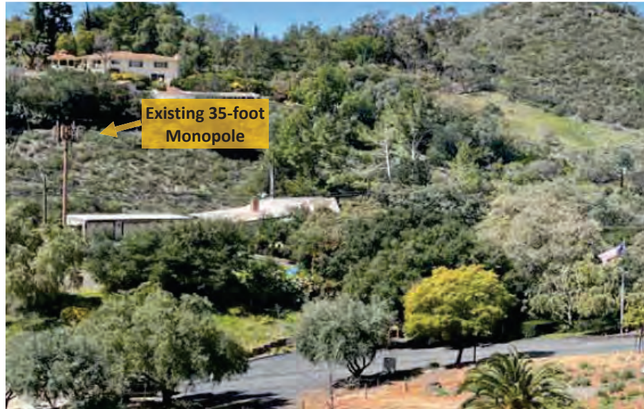
Figure 1: Existing 45-foot-tall monopole looking west toward the site.
