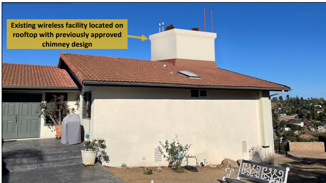
Figure 1: Existing 27-foot-tall wireless facility above the single-family residence looking west toward the site.
