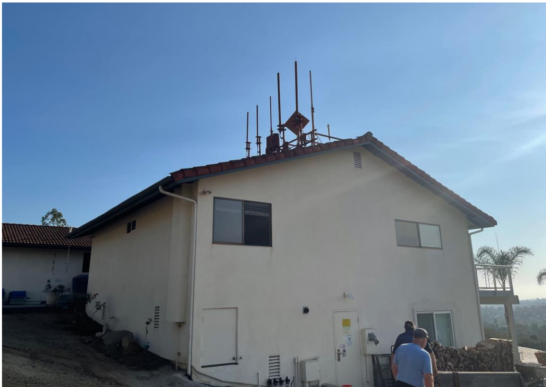
View South toward site and equipment room – Cupola permitted (not installed)
